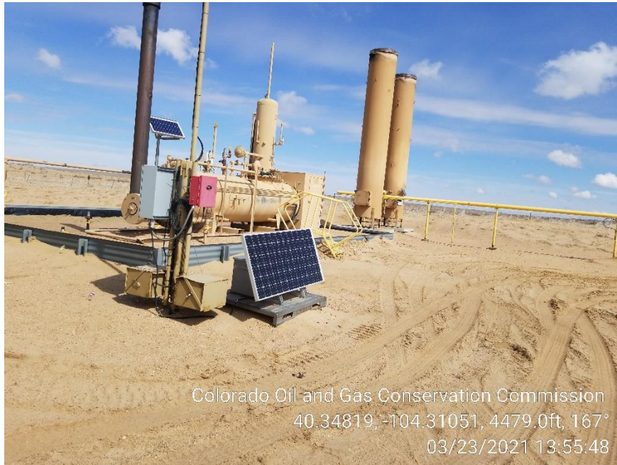
Photo 3 – Separator and ECDs
