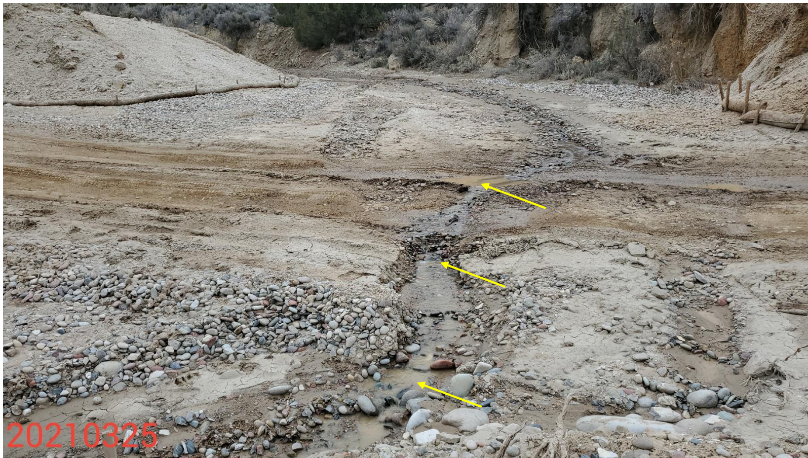
Photo 15: Continued from photo 14. Photo shows headcutting/degradation evident within the stream crossing. Photo also shows sediment discharge into the stream/waters of the state occurring at the stream crossing.
