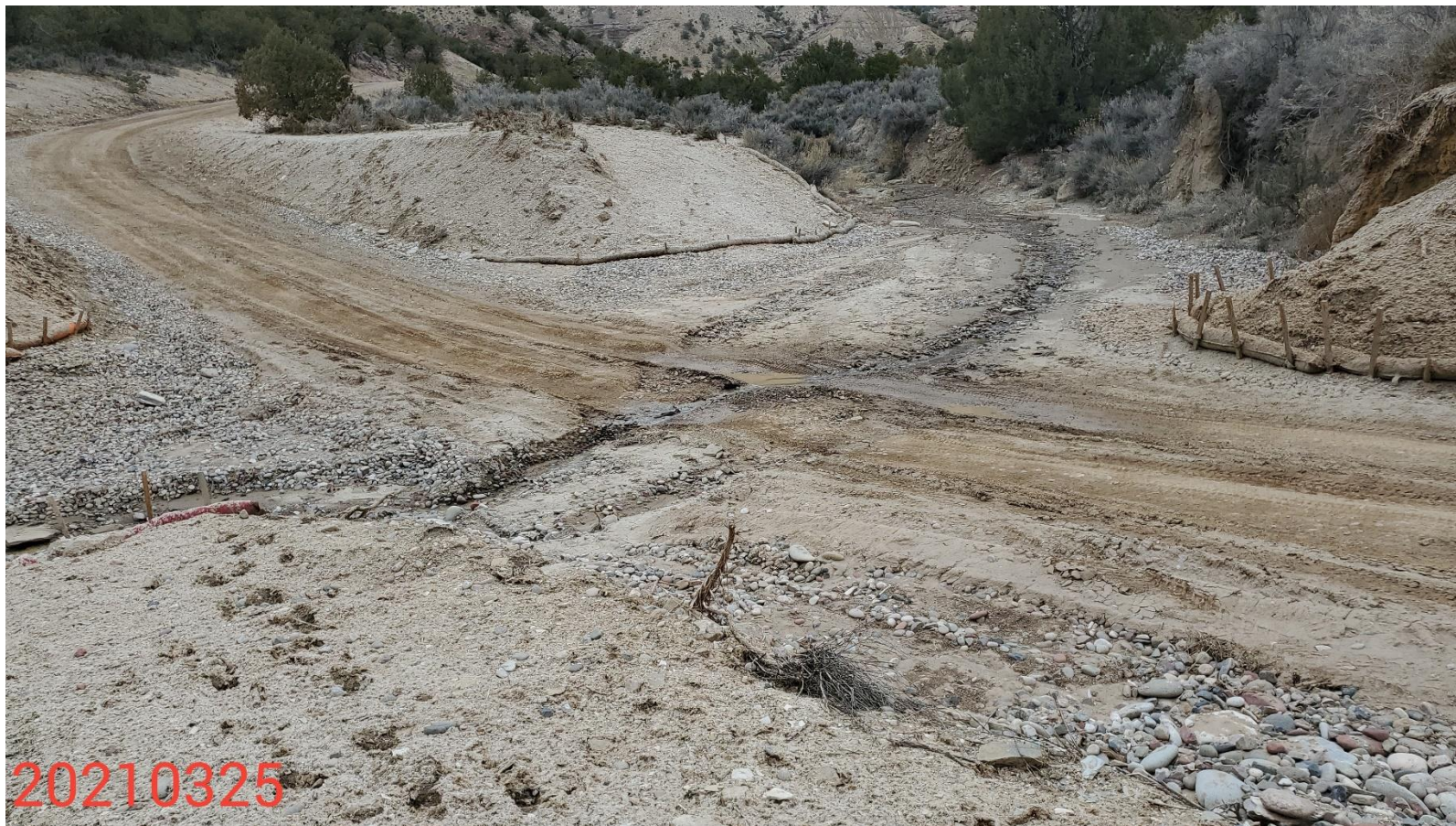
Photo 14: Photo taken from the access road at the stream crossing, facing north. Photo shows proper BMPs per good engineering practices remain missing, or insufficient to stabilize access road at stream crossing, and protect stream/waters of the state; Head cutting and sediment laden discharge observed.
