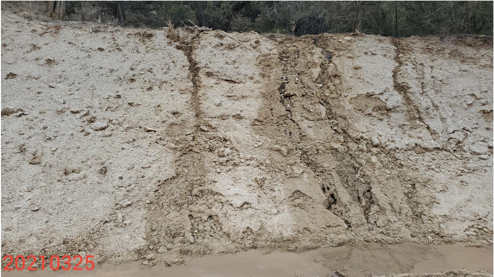
Photo 10: Photo taken from the cut slopes on the west end of the Location. Photo shows that control measures to properly manage run-on, and to stabilize protect the slopes of the Location remain missing, insufficient or inadequate. Sediment has filled the ditch.
