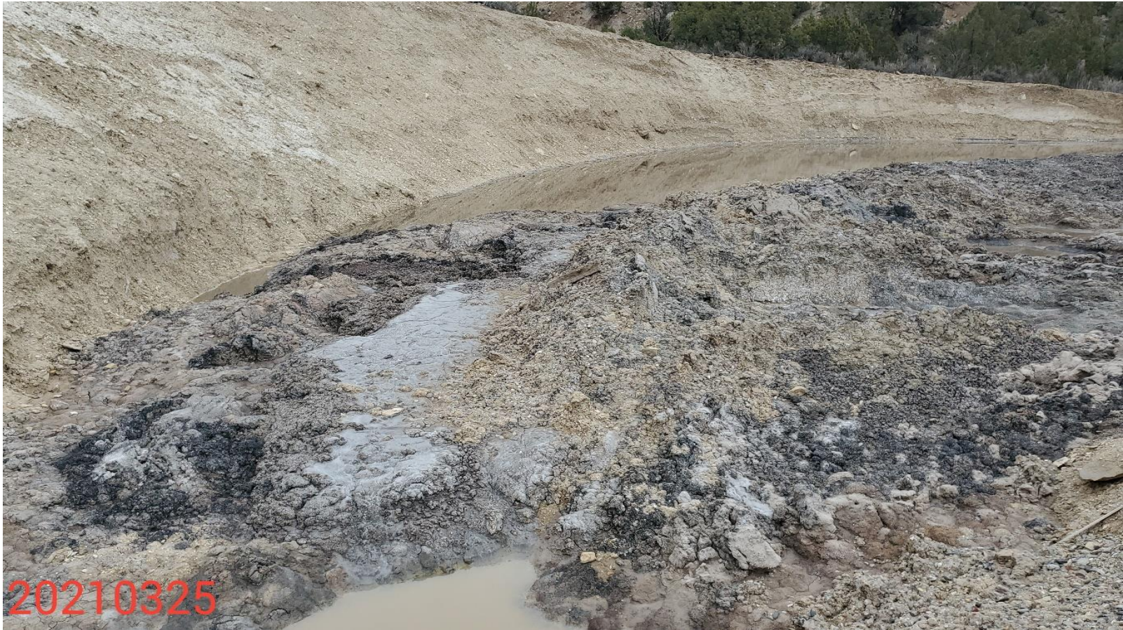
Photo 6: Photo taken from the northwest end of the Location, facing northeast. Photo shows drill pit. Interim reclamation of the Location due; pit will require closure in accordance with 900 series rules.
