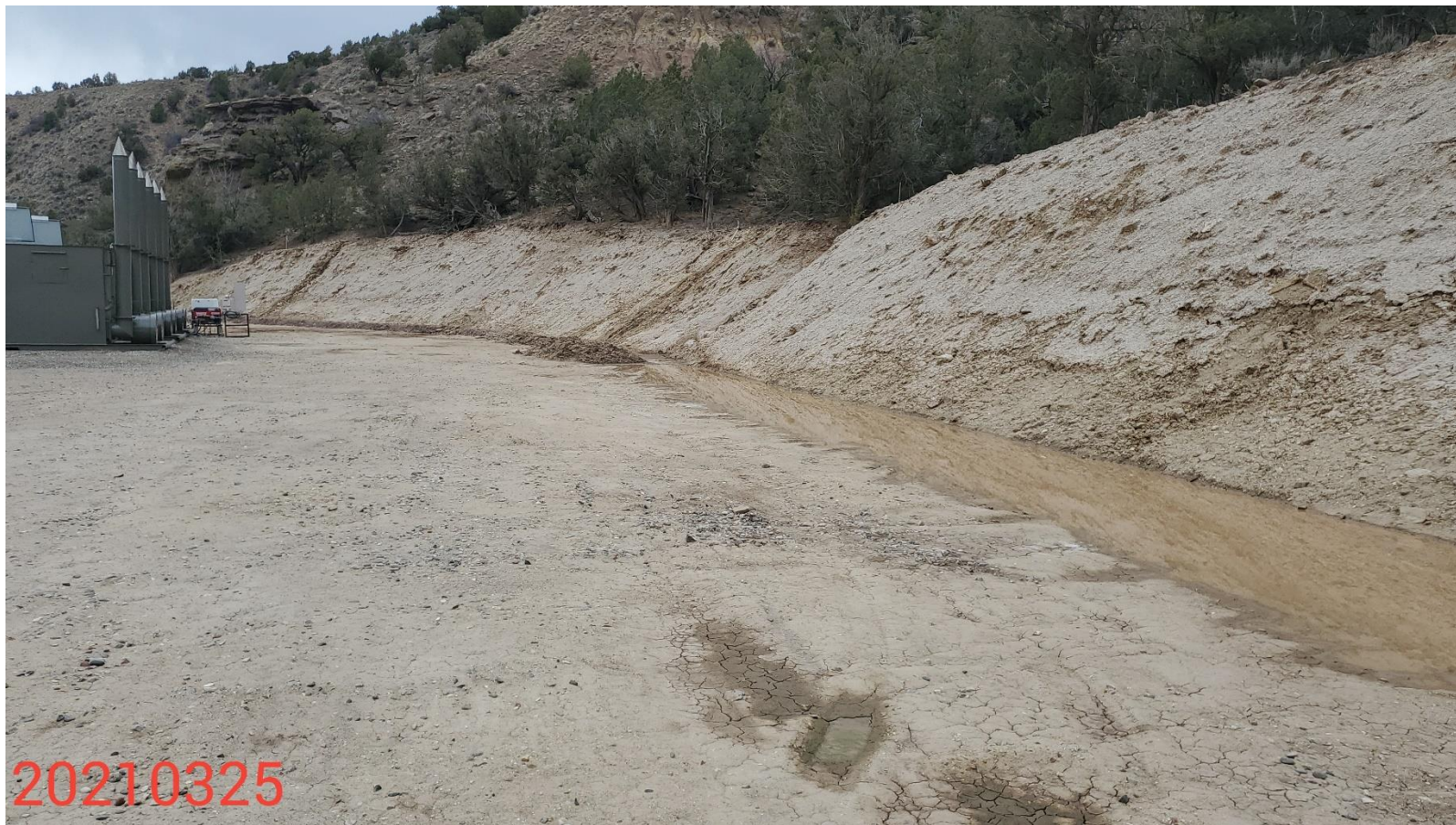
Photo 7: Photo taken from the northwest end of the Location, facing south. Photo shows stormwater ditch on the west end of the pad has filled with sediment, and is no longer in proper functioning condition. Photo also shows that a berm has been installed along a portion of the ditch.
