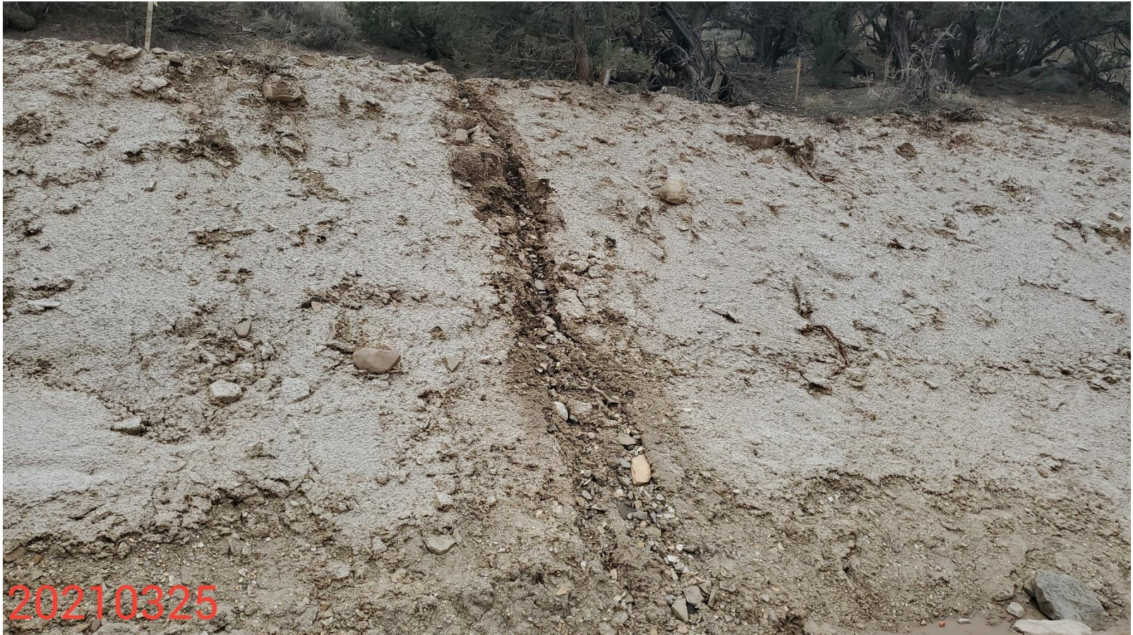
Photo 11: Photo taken from the cut slopes on the west end of the Location. Photo shows that control measures to properly manage run-on, and to stabilize protect the slopes of the Location remain missing, insufficient or inadequate.
