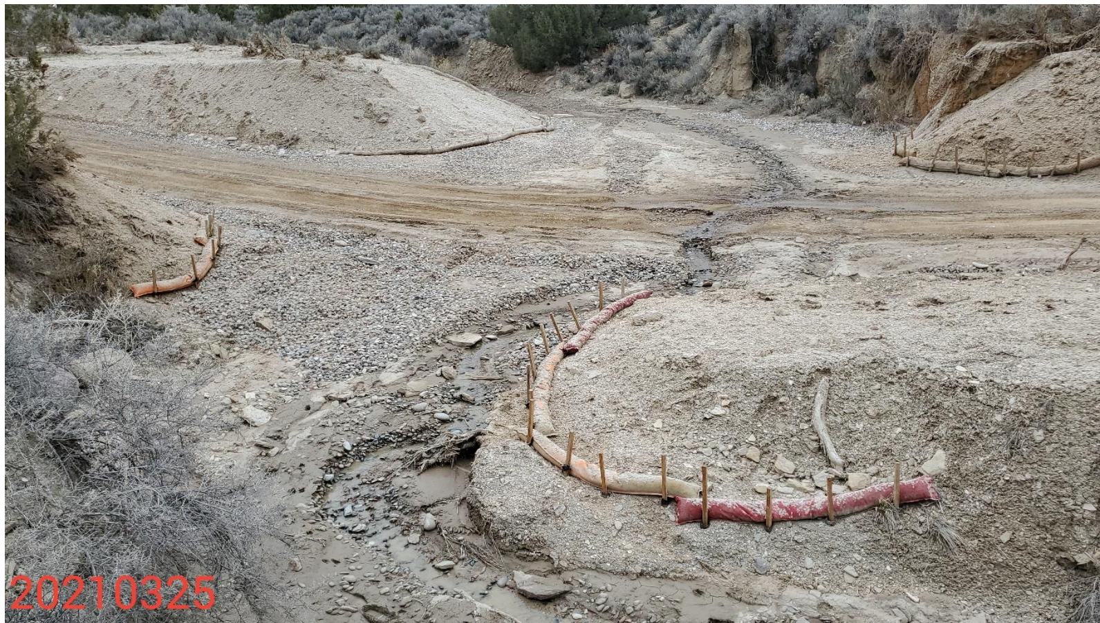
Photo 19: Photo taken from below the stream crossing, facing upstream. Photo shows headcutting/degradation evident within the stream crossing. Photo also shows sediment discharge into the stream/waters of the state occurring at the stream crossing.
