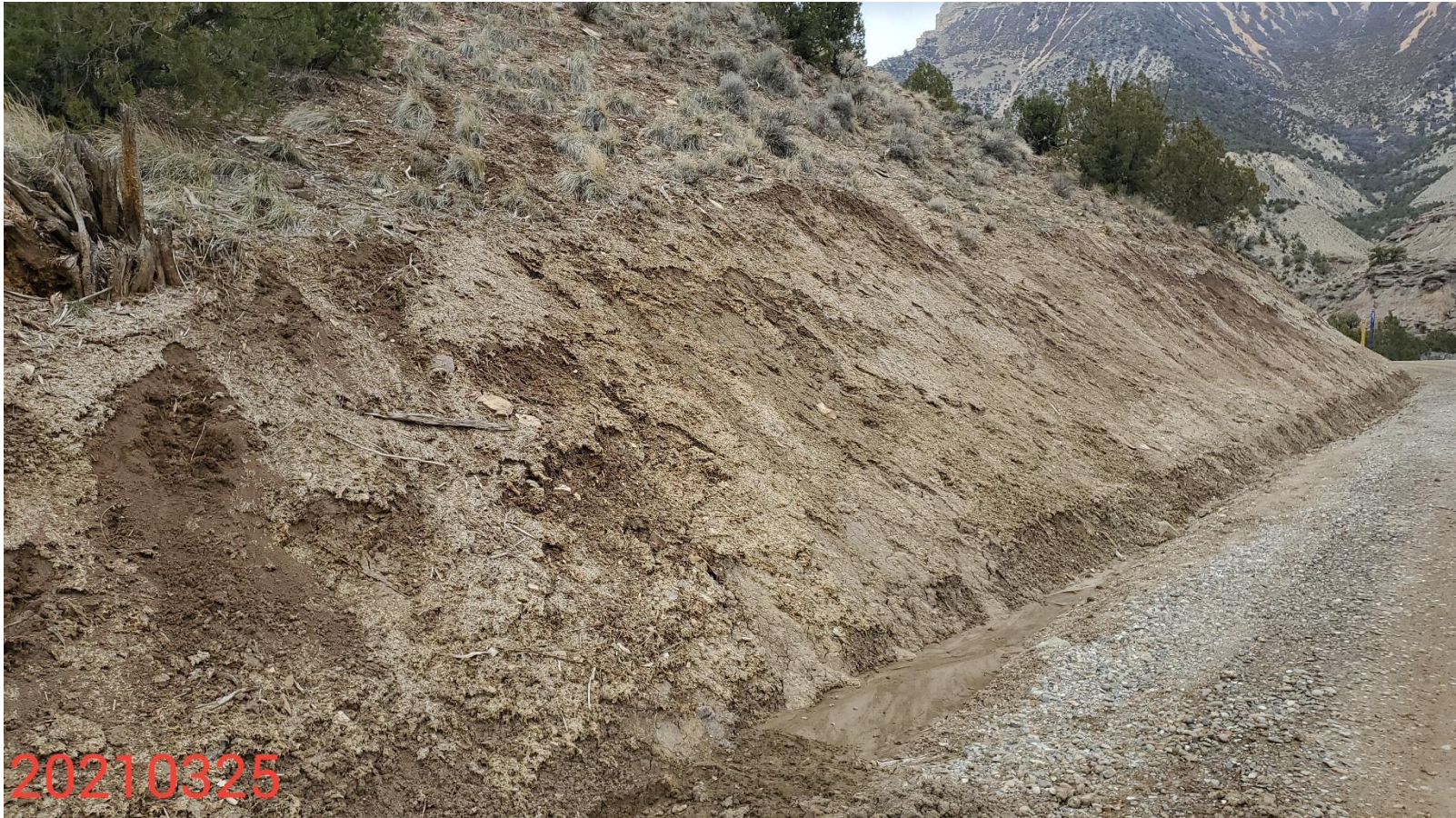
Photo 13: Photo taken from the access road south of the Location, facing north. Photo shows that the hydromulch applied to the slopes are degrading, and are no longer in proper functioning condition. Degradation evident. BMP alone insufficient to manage run-on and stabilize/protect slopes.
