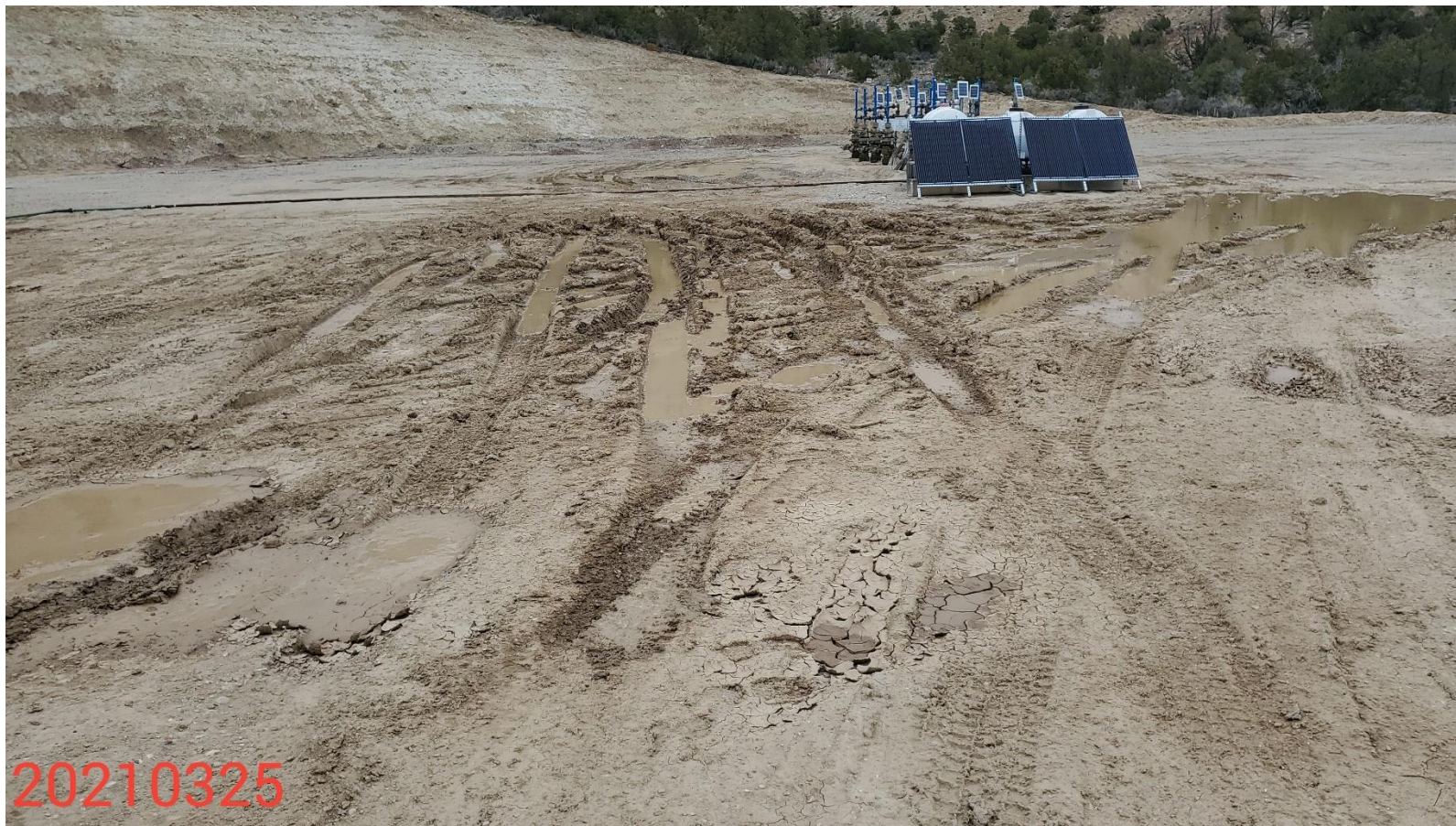
Photo 12: Photo taken from the Location, facing north. Photo shows control measures to stabilize/protect unpaved areas of the Location are missing or insufficient
