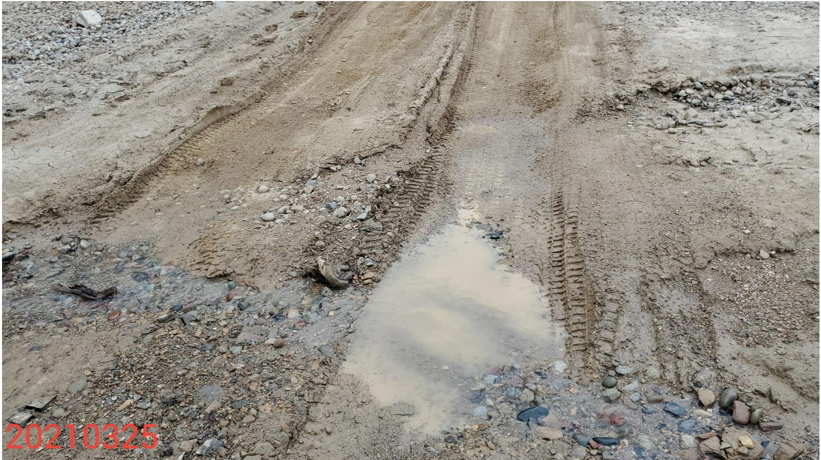
Photo 18: Photo shows headcutting/degradation evident within the stream crossing. Photo also shows sediment discharge into the stream/waters of the state occurring at the stream crossing.
