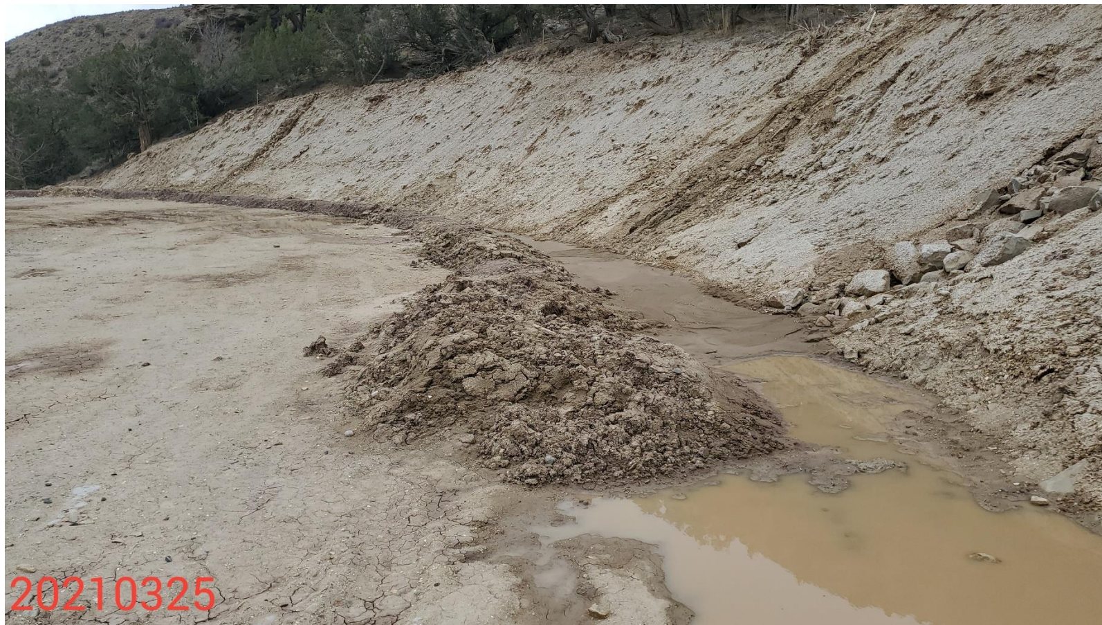
Photo 8: Photo taken from the west end of the Location, facing south. Photo shows stormwater ditch on the west end of the pad has filled with sediment, and is no longer in proper functioning condition. Photo also shows that a berm has been installed along a portion of the ditch; berm has not been installed in accordance with good engineering practices; berm has not been properly compacted.
