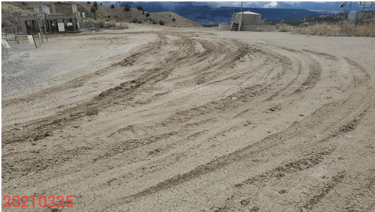
Photo 3: Photo taken from the north end of the Location, facing southeast. Photo shows that control measures to stabilize/protect unpaved areas of the Location are missing or insufficient.
