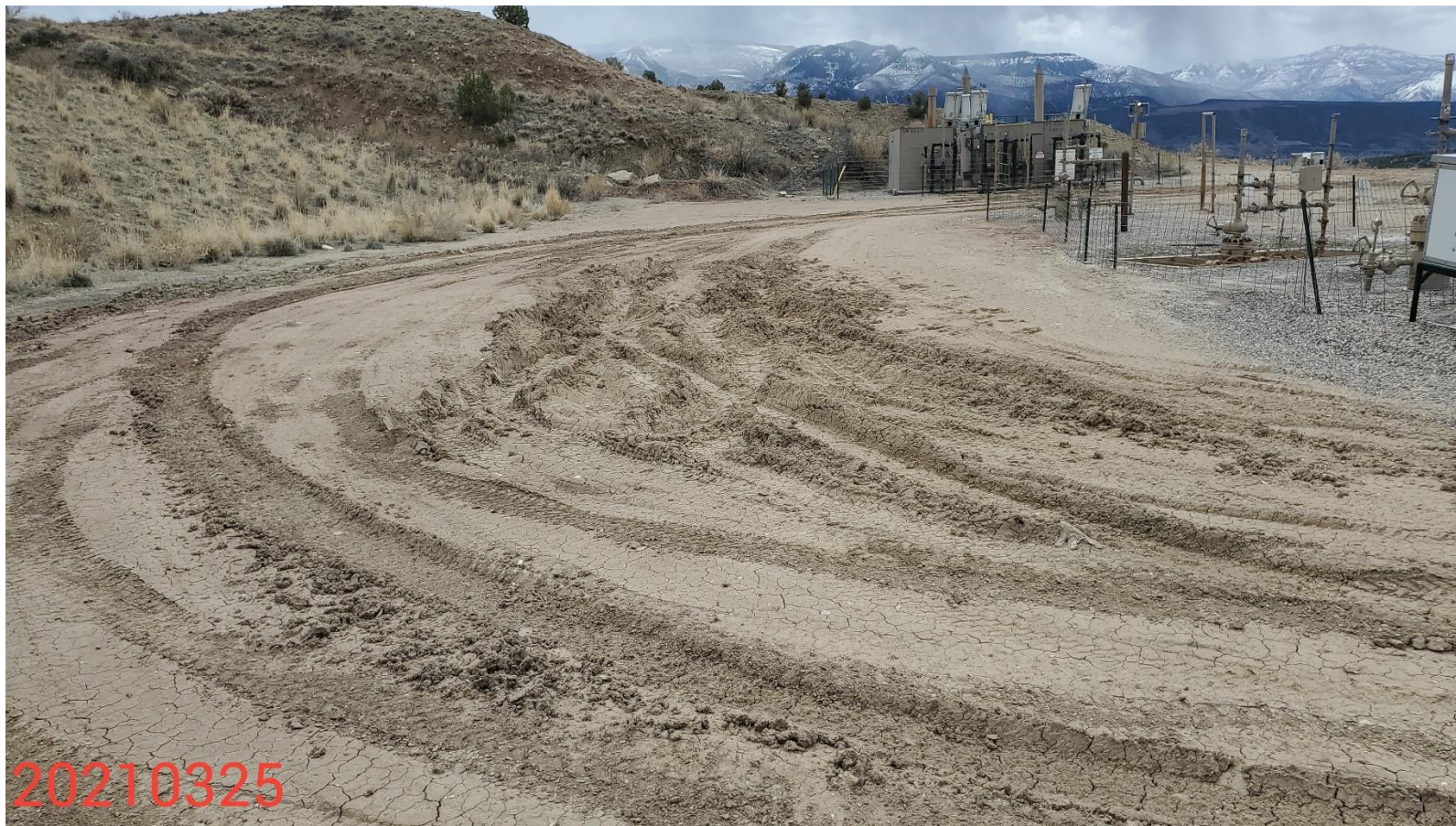
Photo 2: Photo taken from the north end of the Location, facing southeast. Photo shows that control measures to stabilize/protect unpaved areas of the Location are missing or insufficient.
