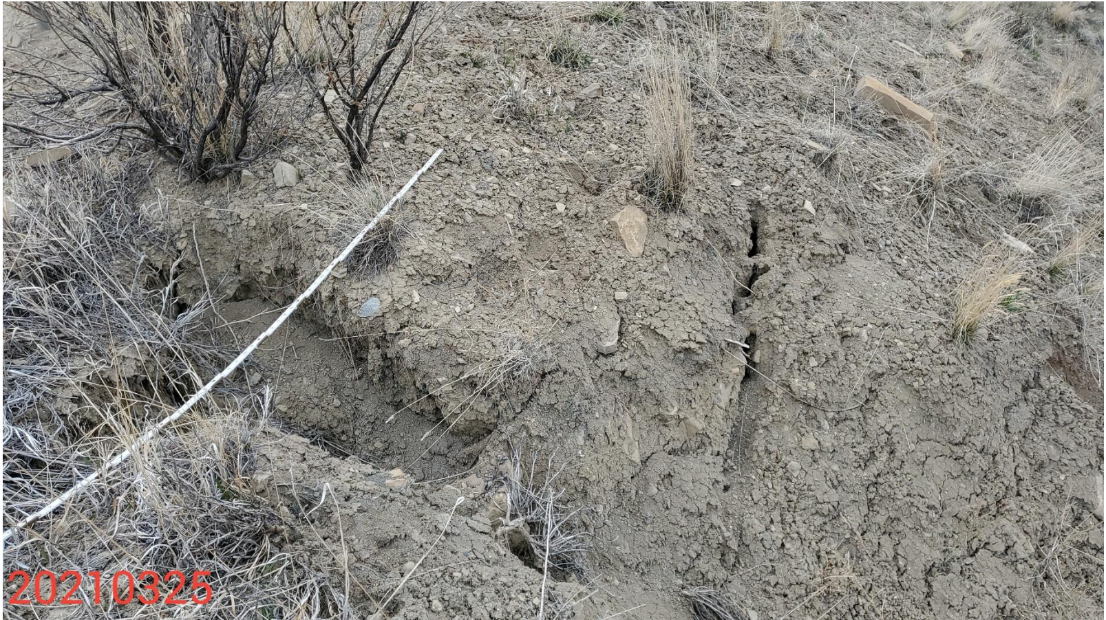
Photo 5: Photo taken from the slopes on the west end of the Location. Photo shows that control measures to stabilize/protect the cut/fill slopes of the Location are missing or insufficient; Gully erosion evident; crack forming within slope. 6 foot measuring stick used for reference.
