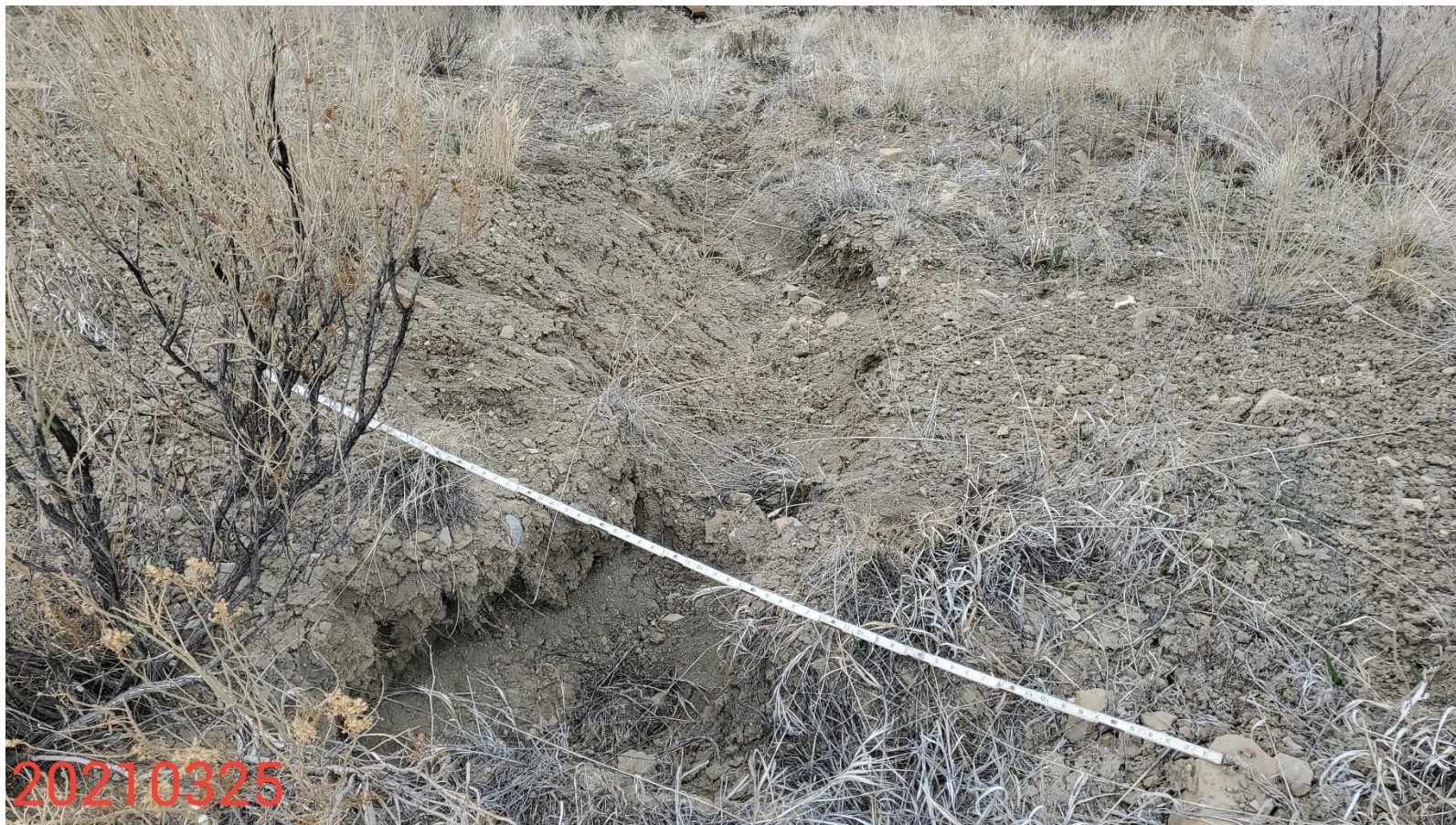
Photo 4: Photo taken from the slopes on the west end of the Location. Photo shows that control measures to stabilize/protect the cut/fill slopes of the Location are missing or insufficient; Gully erosion evident; crack forming within slope. 6 foot measuring stick used for reference.
