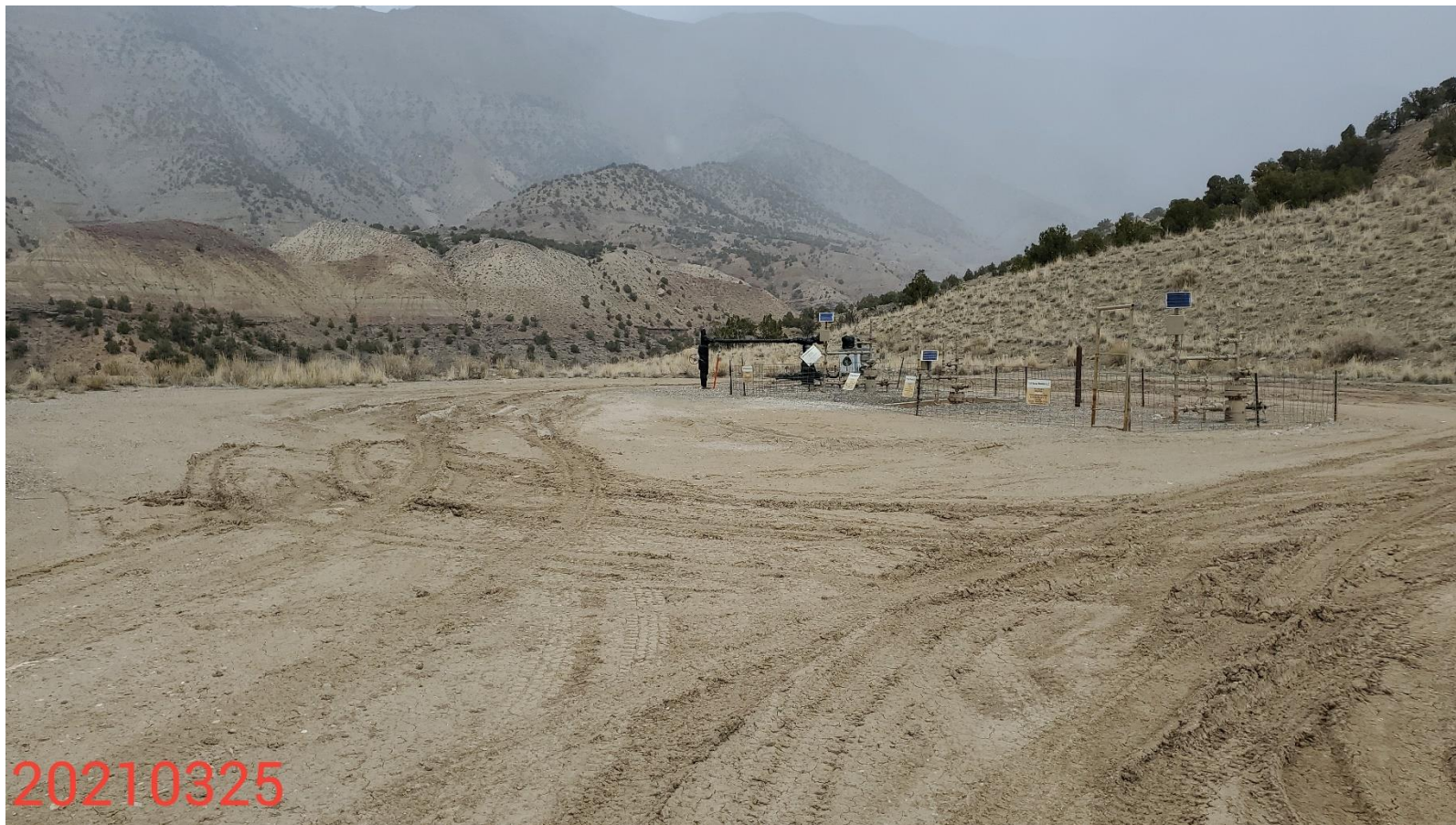
Photo 1: Photo taken from the south end of the Location, facing north. Photo shows that control measures to stabilize/protect unpaved areas of the Location are missing or insufficient.
