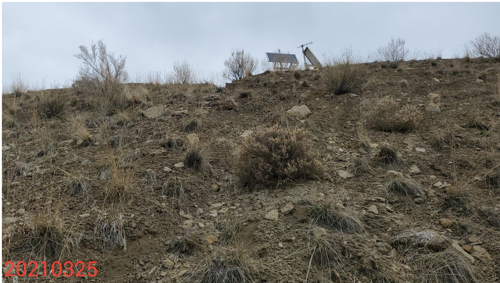
Photo 6: Photo taken from the slopes on the west end of the Location. Photo shows that control measures to stabilize/protect the cut/fill slopes of the Location are missing or insufficient; Gully erosion evident; crack forming within slope.
