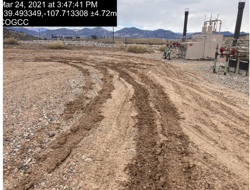
Lack of stabilization/compaction
