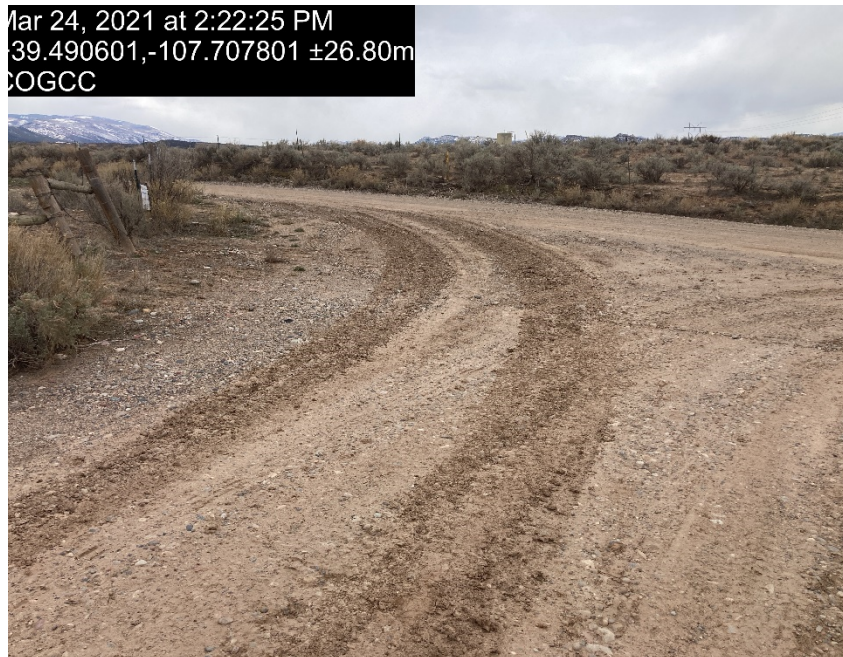
Lack of stabilization/compaction
