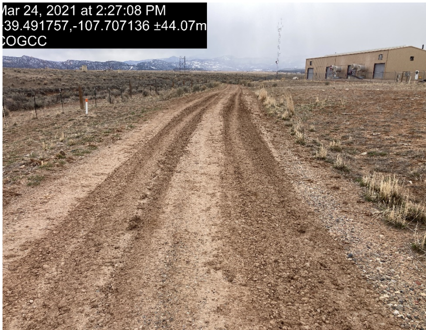
Lack of stabilization/compaction
