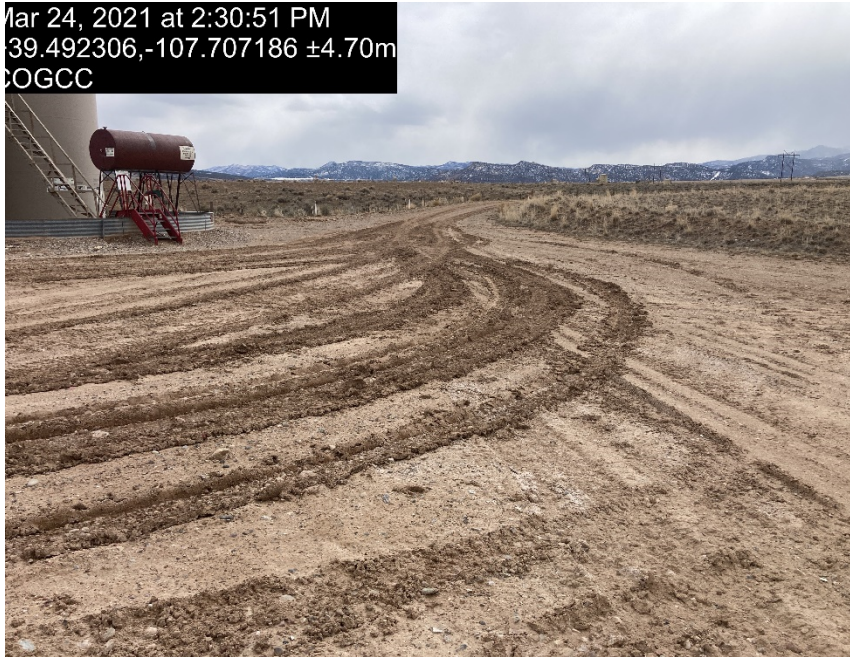
Lack of stabilization/compaction
