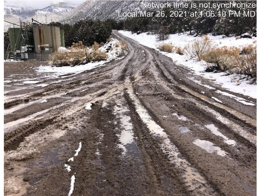
Photo #3316 No form of tracking control at entrance to location.
