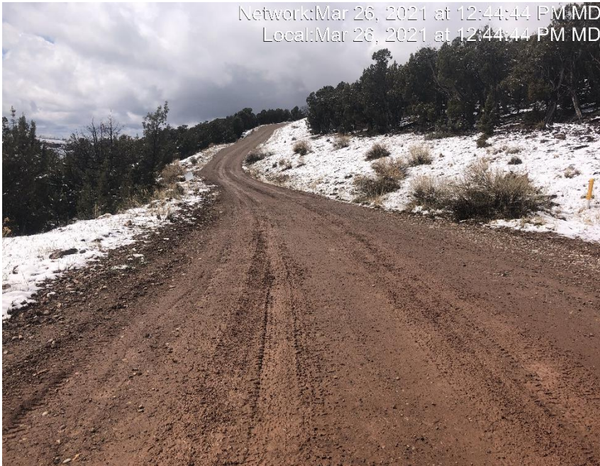
Photo #3310 No form of tracking control at entrance to location.
