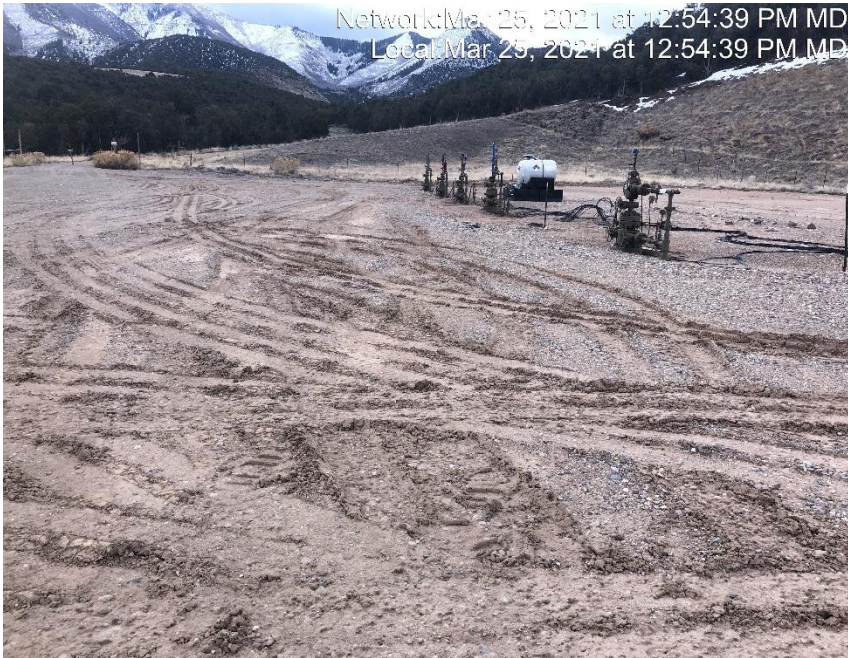
Photo #3278 Location lacks stabilization.
