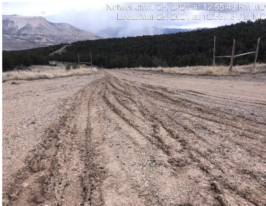
Photo #3280 No form of tracking control at entrance to location
