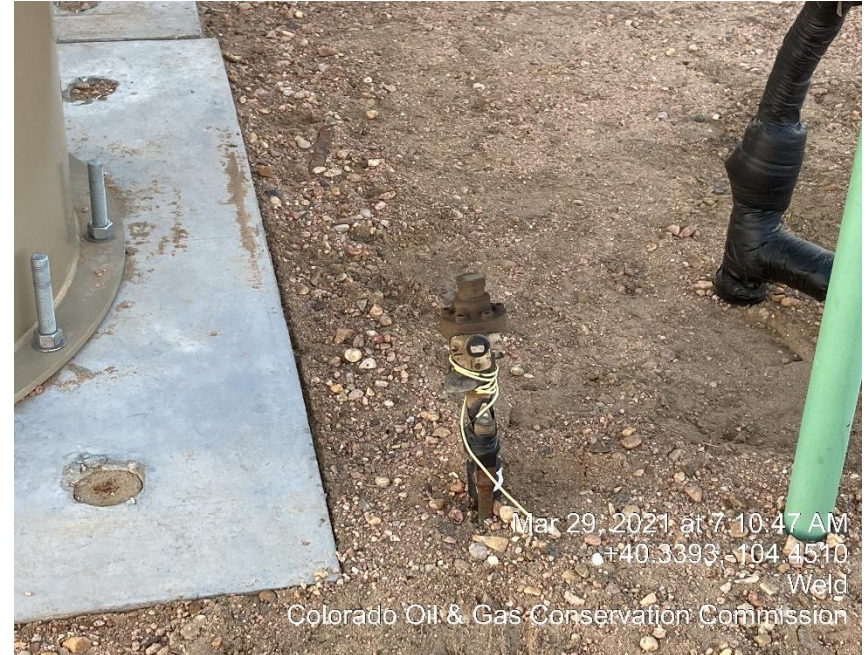
Photo #2 Unmarked Riser
