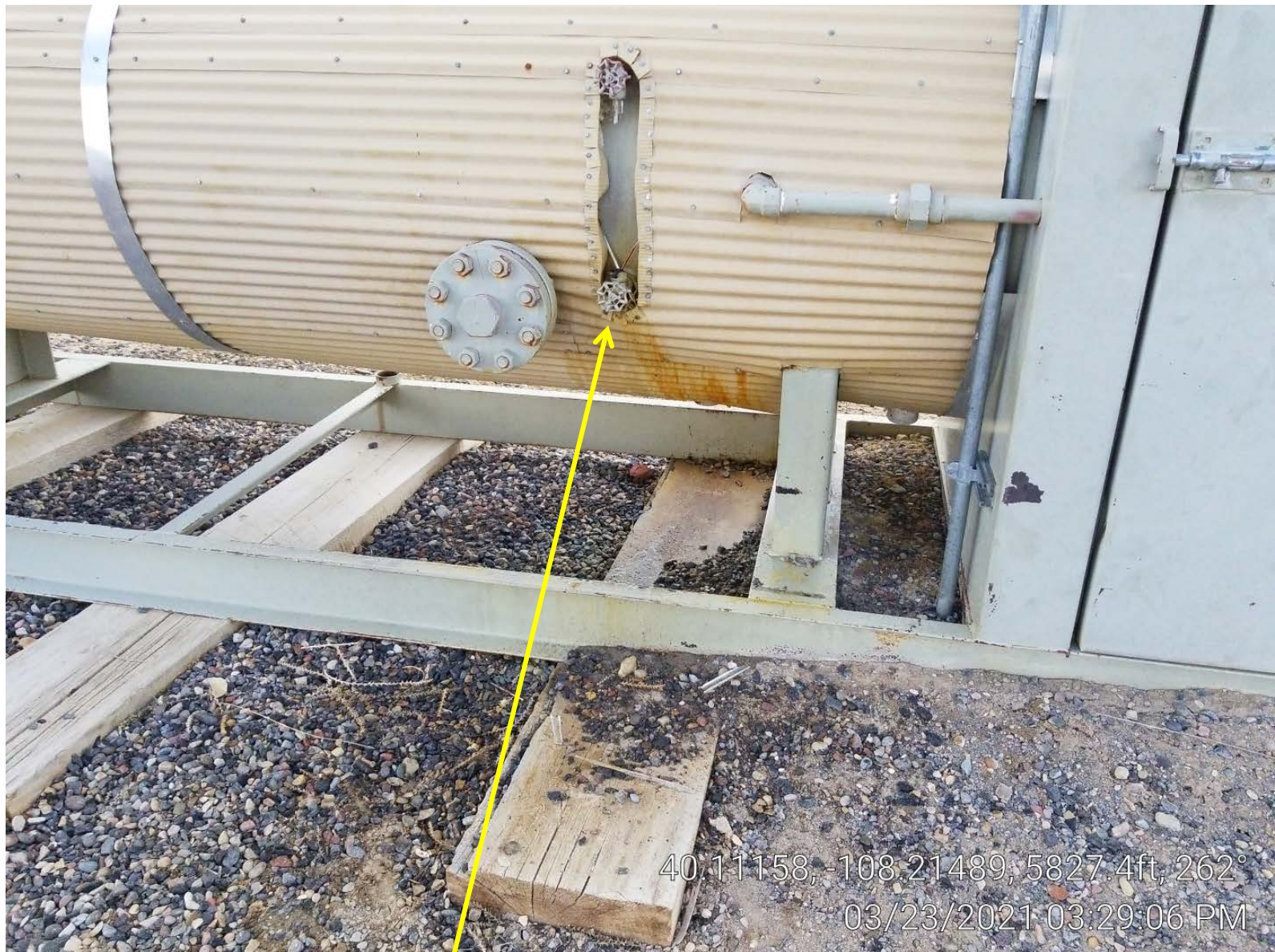
Photo 5. Leaking lower valve of cracked sight glass closed by inspector.
