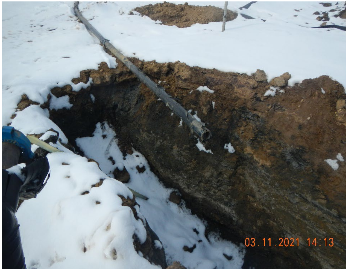
Photo #7 flowline to wellhead.
