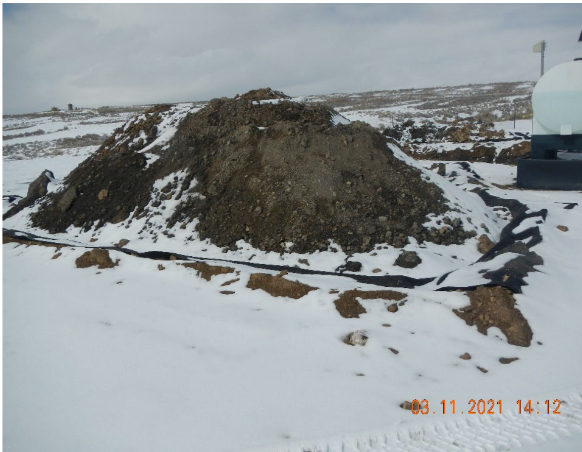
Photo #2 stockpiled soil from spill excavation.
