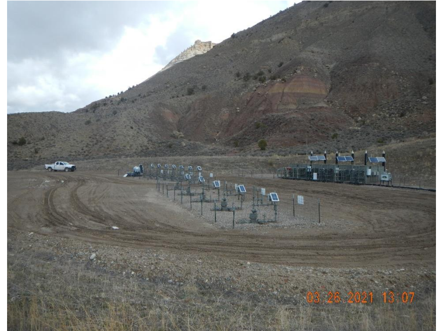
Location shows signs of lack of stabilization
