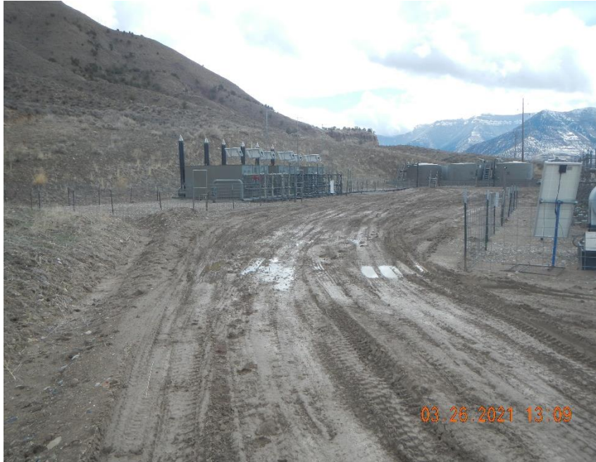
Location shows signs of lack of stabilization
