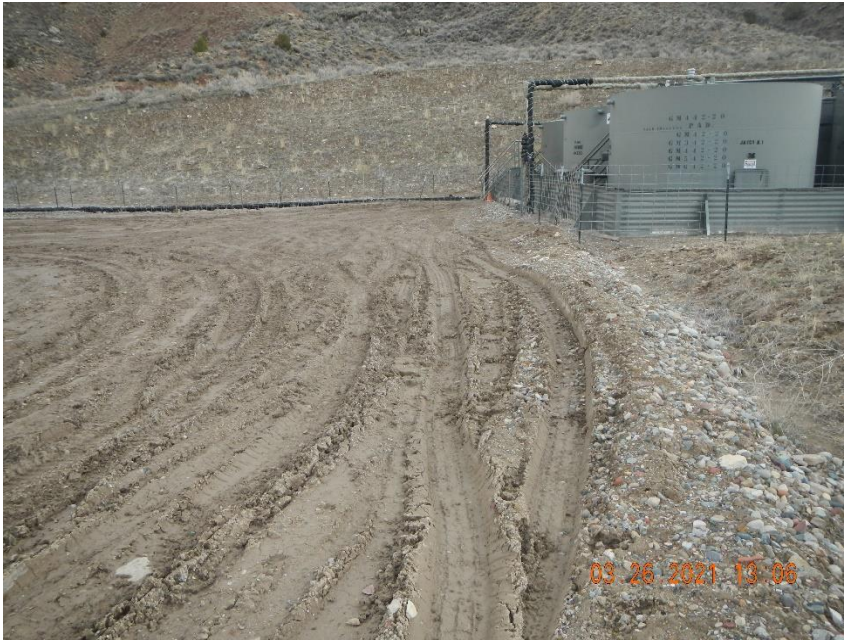
Location shows signs of lack of stabilization
