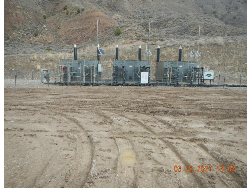
Location shows signs of lack of stabilization
