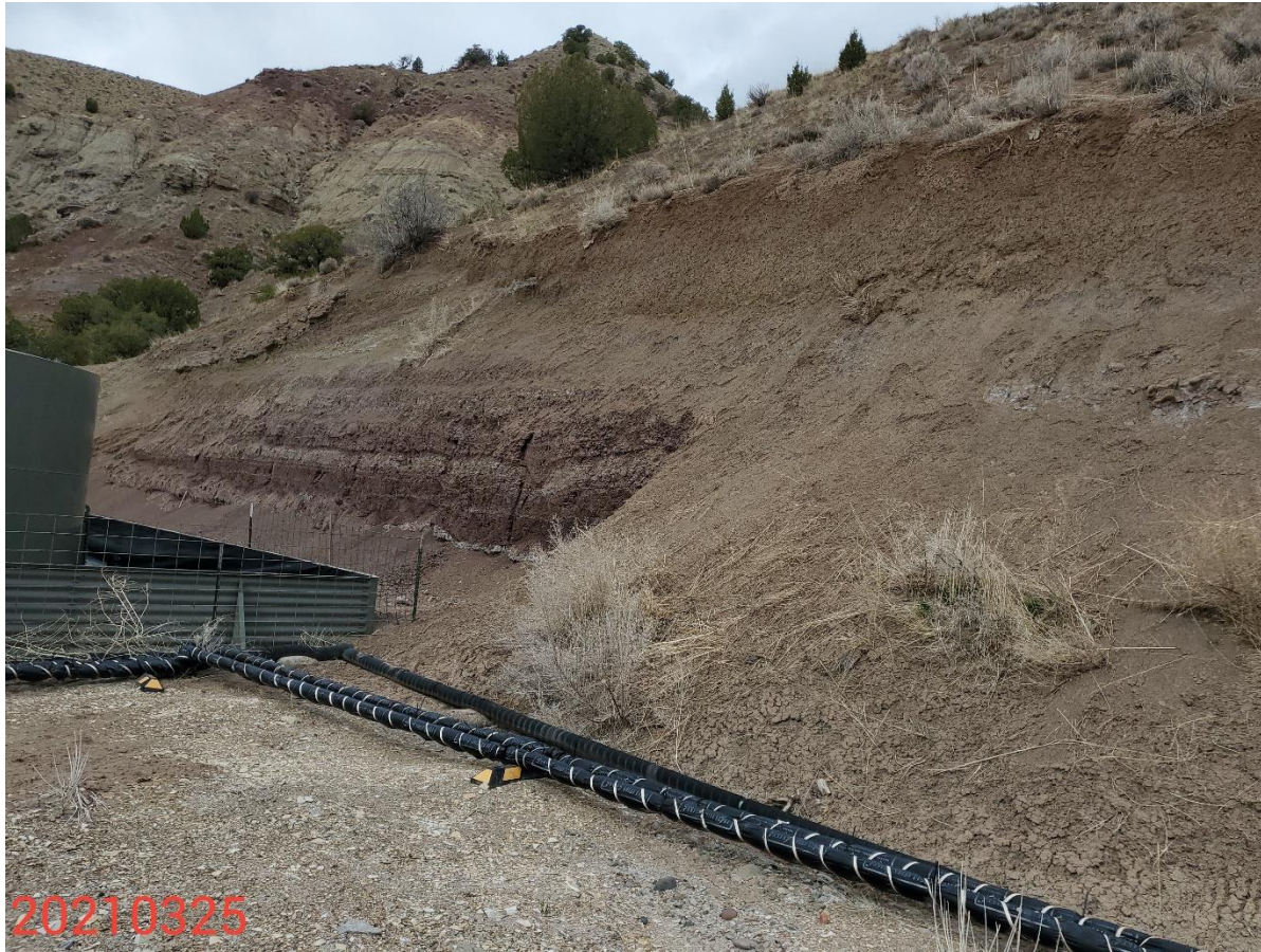
Photo 5: Photo taken from the north end of the Location. Photo shows that control measures to protect/stabilize the cut slopes on the Location remain missing or insufficient.
