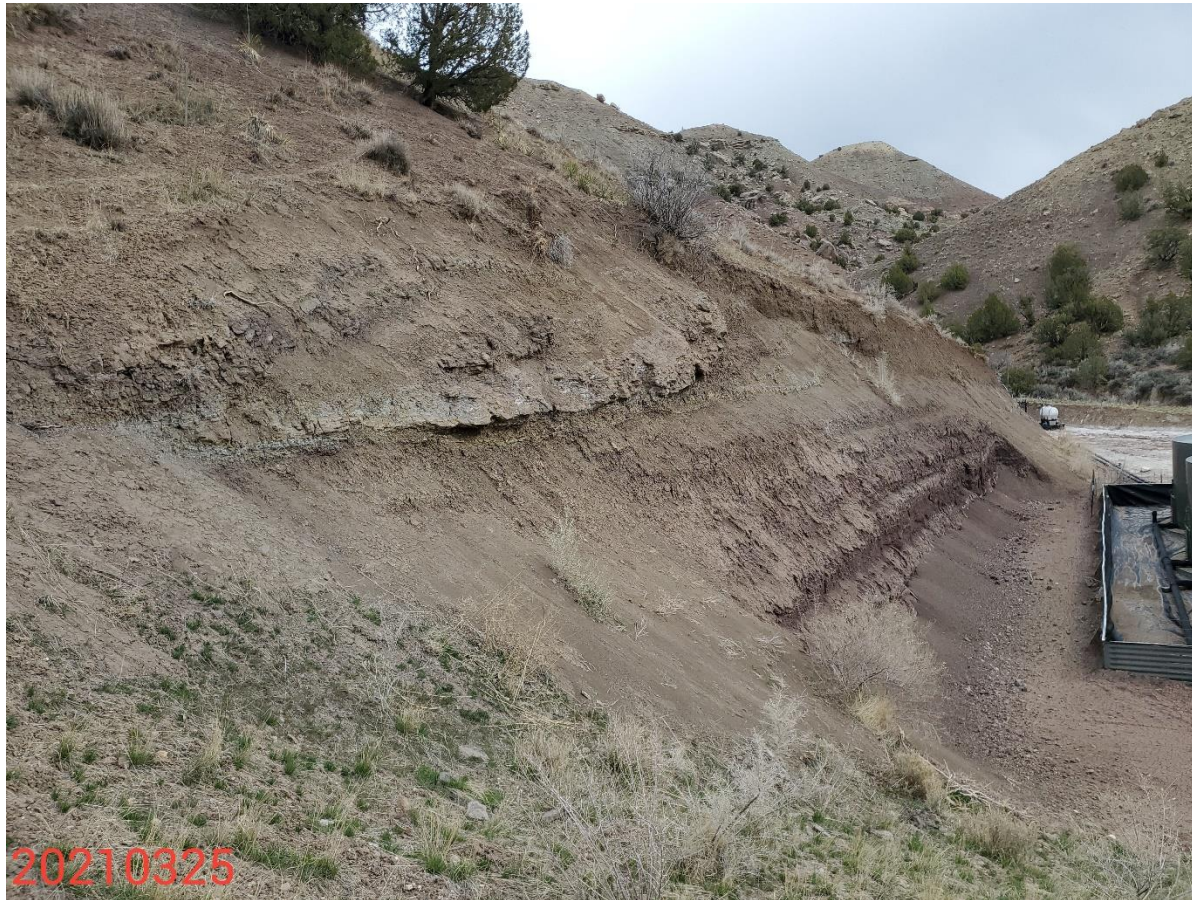
Photo 9: Photo taken from the north end of the Location. Photo shows that control measures to protect/stabilize the cut slopes on the Location remain missing or insufficient.
