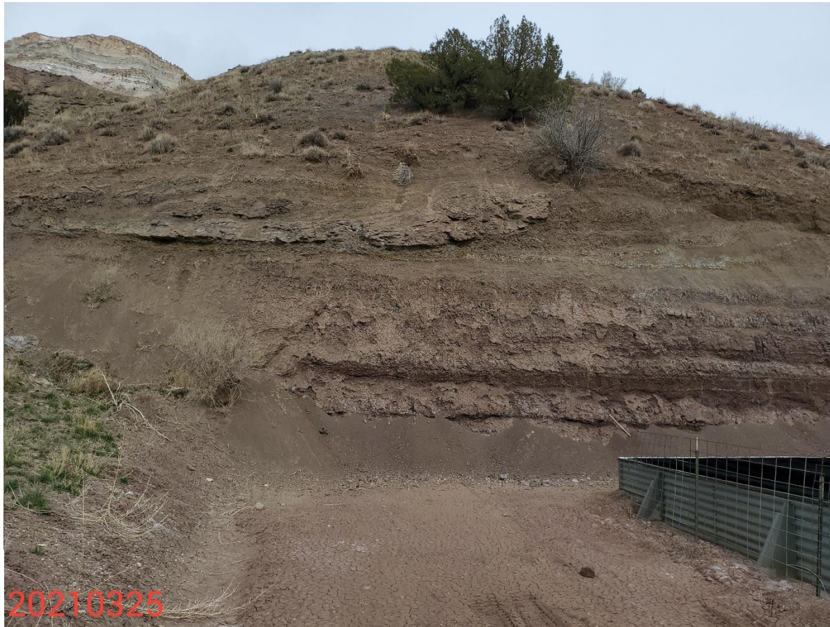
Photo 8: Photo taken from the north end of the Location. Photo shows that control measures to protect/stabilize the cut slopes on the Location remain missing or insufficient.
