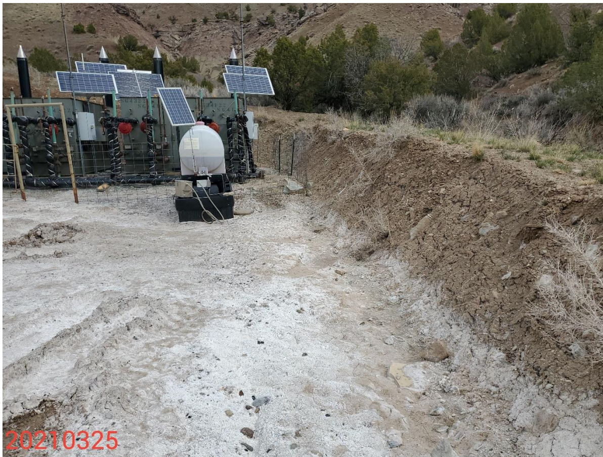
Photo 7: Photo taken from the north end of the Location. Photo shows that control measures to protect/stabilize the cut slopes on the Location remain missing or insufficient.
