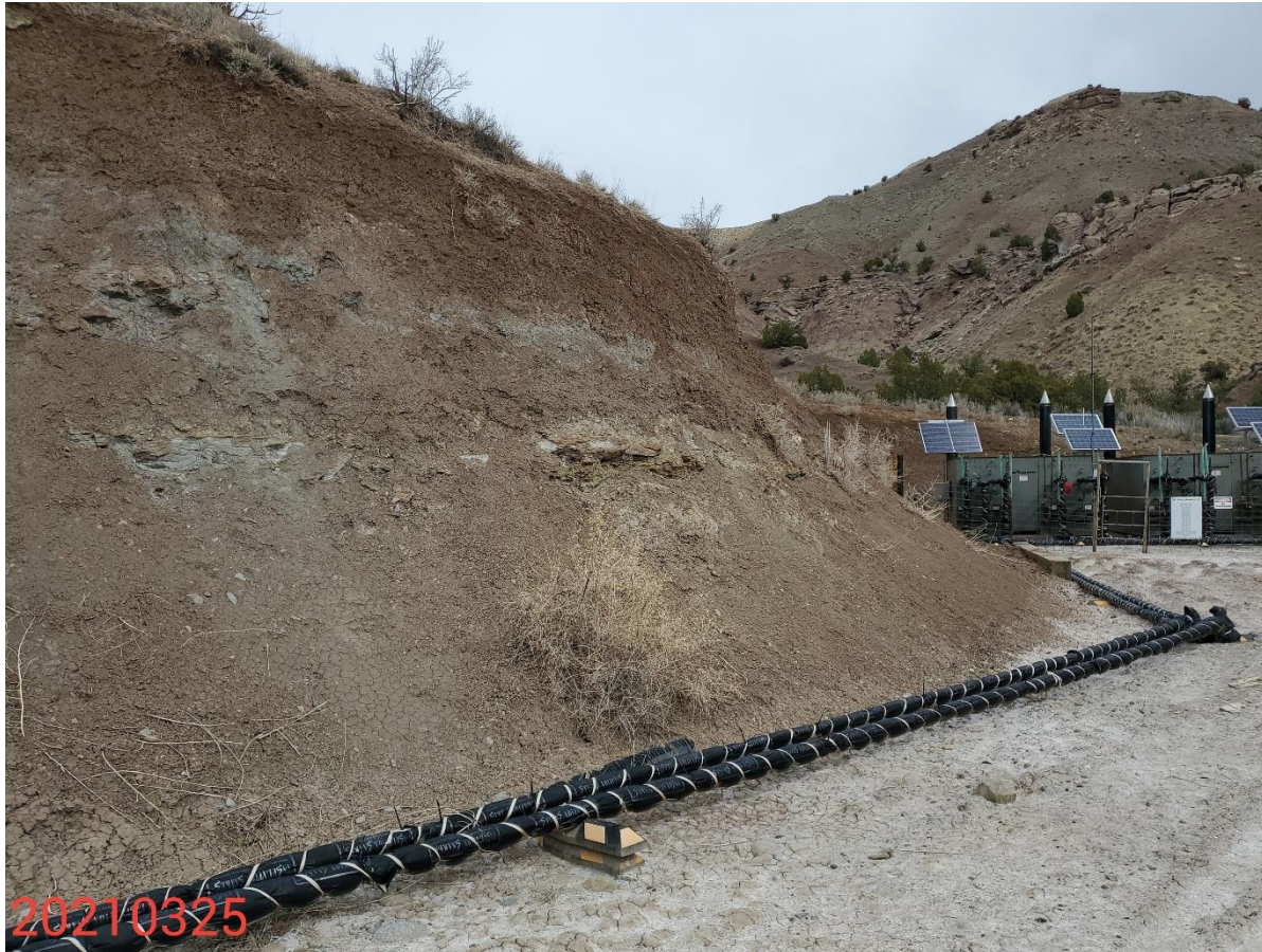
Photo 6: Photo taken from the north end of the Location. Photo shows that control measures to protect/stabilize the cut slopes on the Location remain missing or insufficient.
