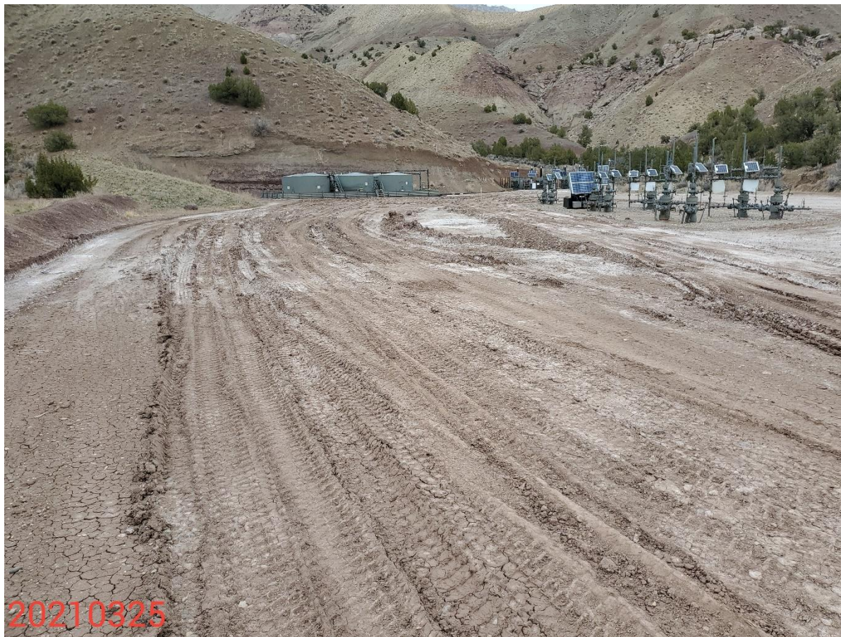
Photo 1: Photo taken from the south end of the Location, facing north. Photos 1-4 show that Pad stabilization concerns remain evident on Location, and appear to have worsened- control measures to stabilize/protect unpaved areas of the Location remain missing or insufficient.
