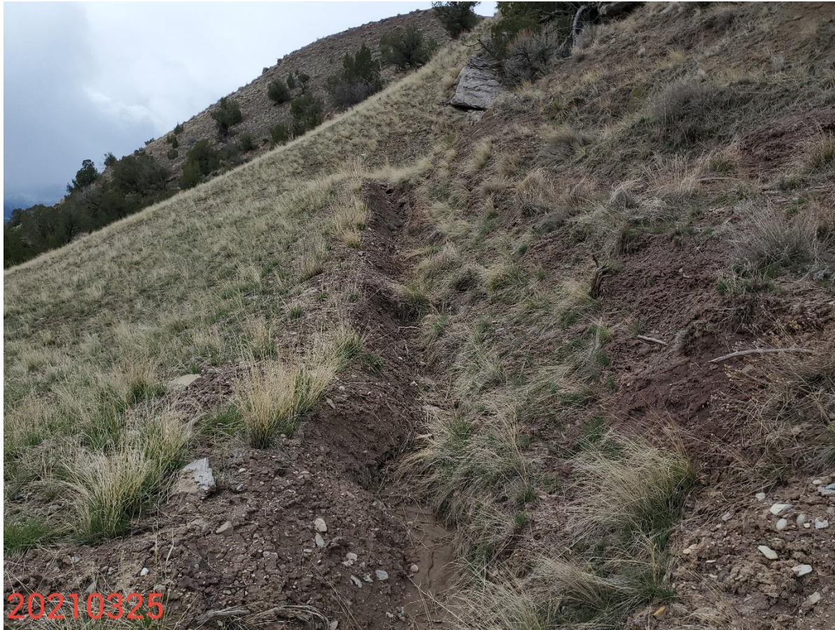
Photo 10: Photo taken from the west end of the Location, facing south. Photo shows stormwater run-on ditch has not been installed in accordance with good engineering practices, or maintained in proper functioning condition; stormwater incision within the ditch evident.
