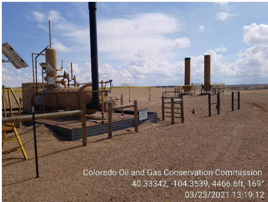
Photo 7 – Separator and ECDs
