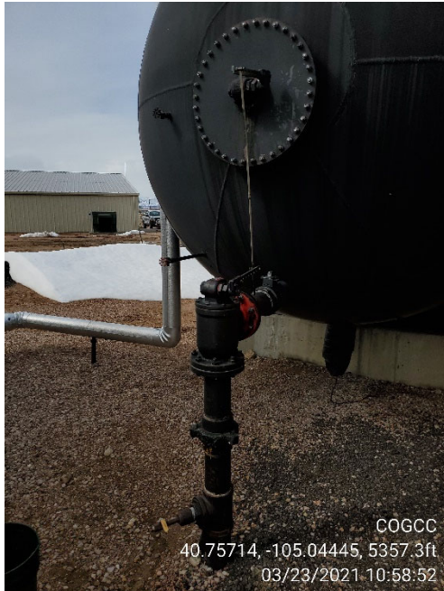
Photo 3: Produced Water sample point on separator at tank battery.
