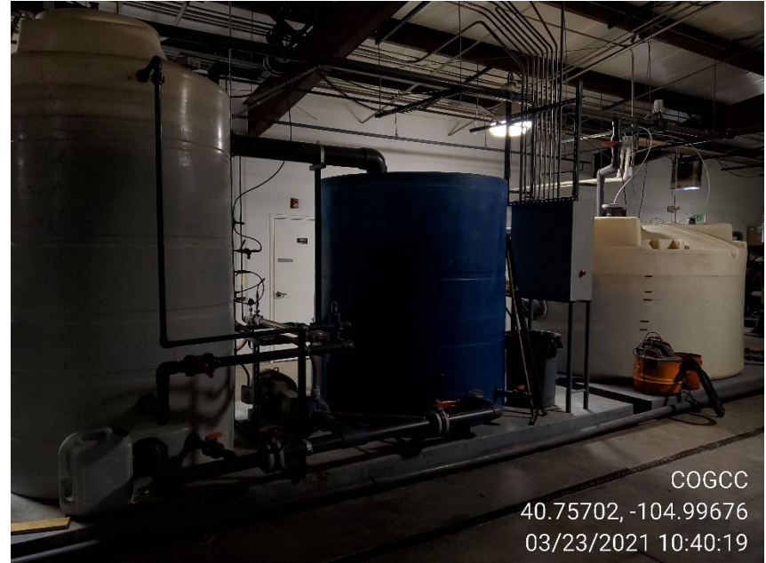
Photo 6: Aeration system and secondary aeration pilot system.
