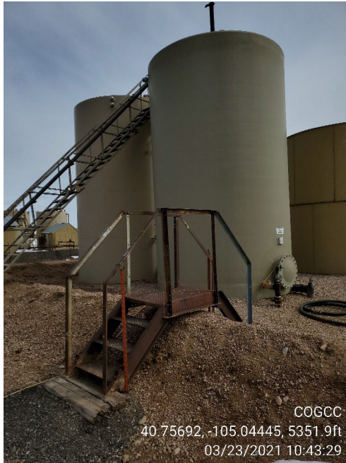
Photo 1: Produced Water ASTs, foreground is aeration tank.
