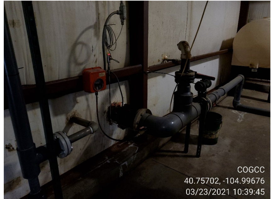
Photo 4: Inflow into treatment building with metering and biocide application.
