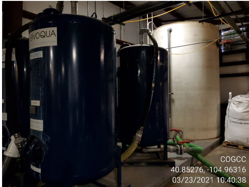
Photo 7: Granulated Activated Carbon filters in foreground and treated water storage tank in background.
