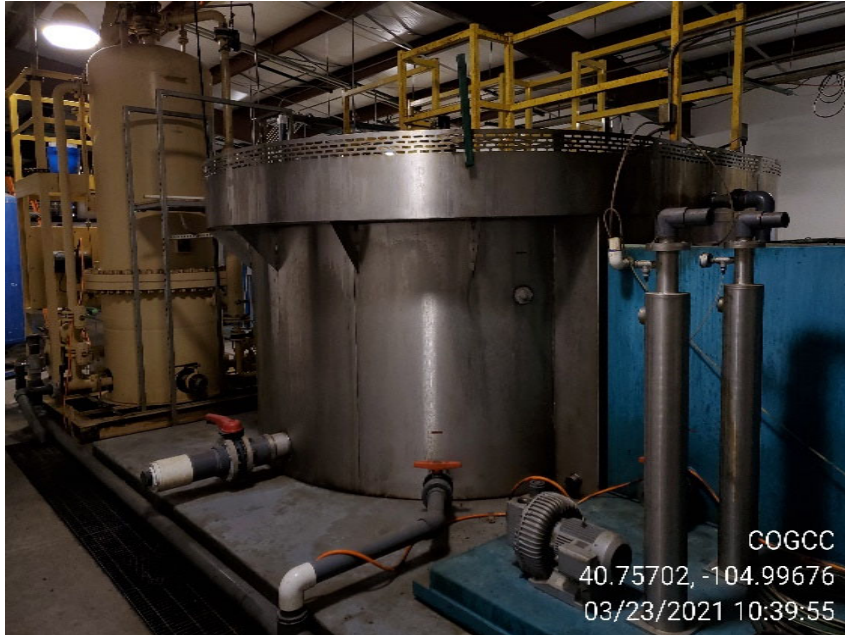
Photo 5: Out of service DAF tank (foreground) used as backwash tank for walnut shell filter. Walnut shell filter is in background.
