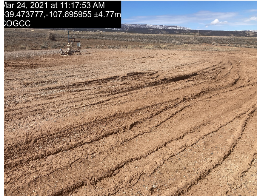
Lack of stabilization / lack of compaction
