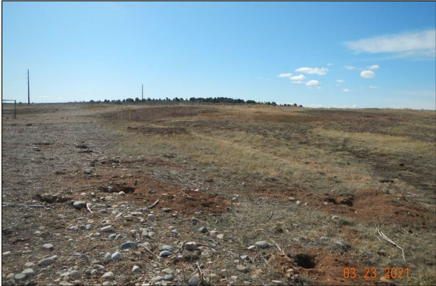
Photo 2. View of the southwestern fill slope facing southeastward from the western corner. Revegetation appears to be progressing in a dormant/grazed condition with crested wheatgrass and western wheatgrass observable.
