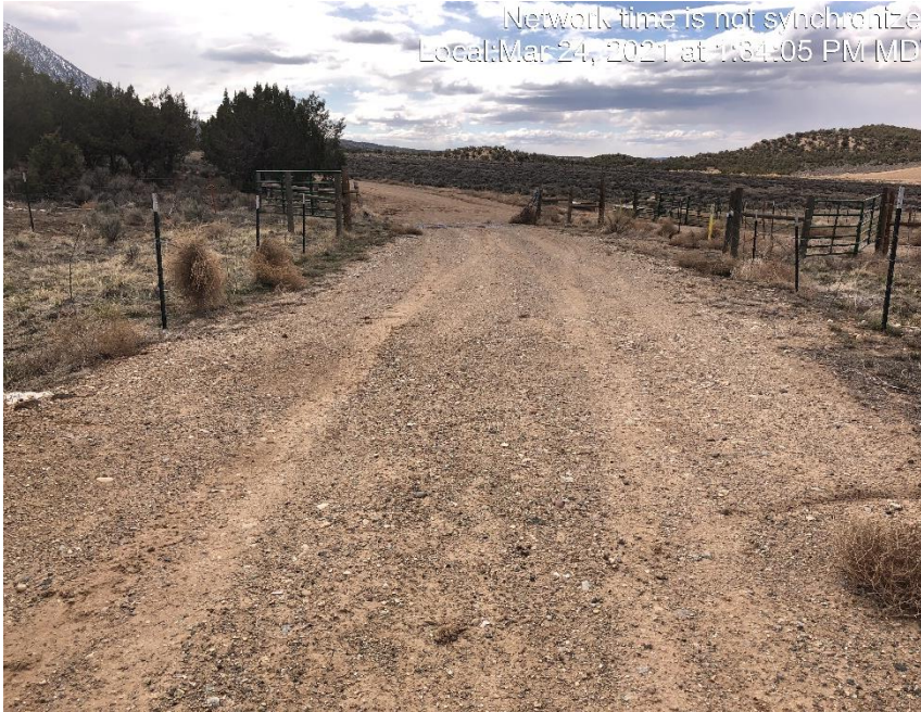
Photo #3270 No form of tracking control at entrance to location.
