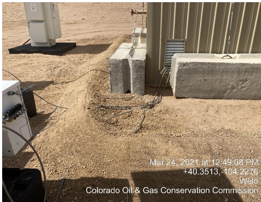
Photo #6 Repaired Berm
