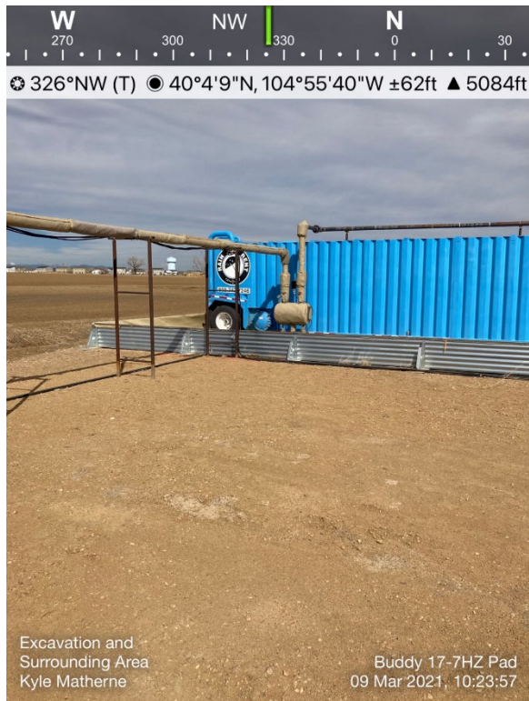
Temporary water tank and containment
