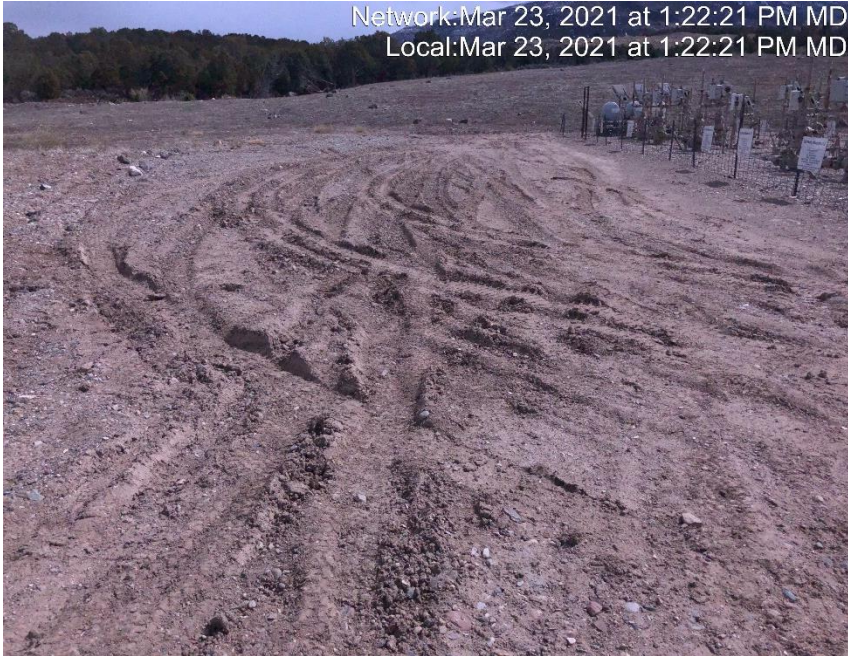
Photo #3254 Location lacks stabilization.
