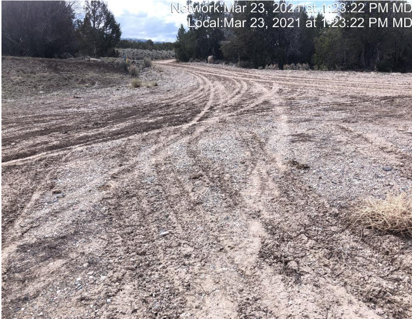
Photo #3256 No form of tracking control at entrance to location
