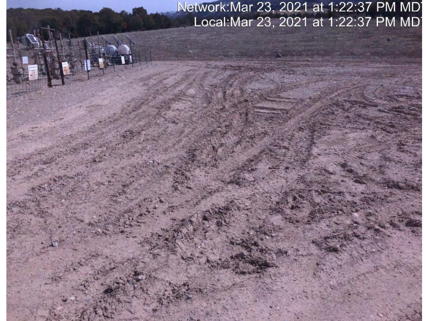
Photo #3255 Location lacks stabilization.
