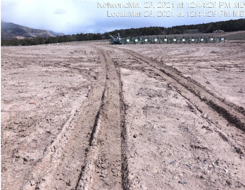
Photo #3242 Location lacks stabilization.
