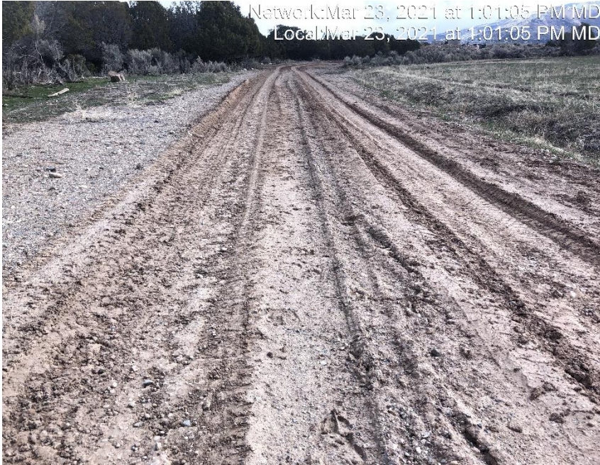
Photo #3251 Access road lacks stabilization
