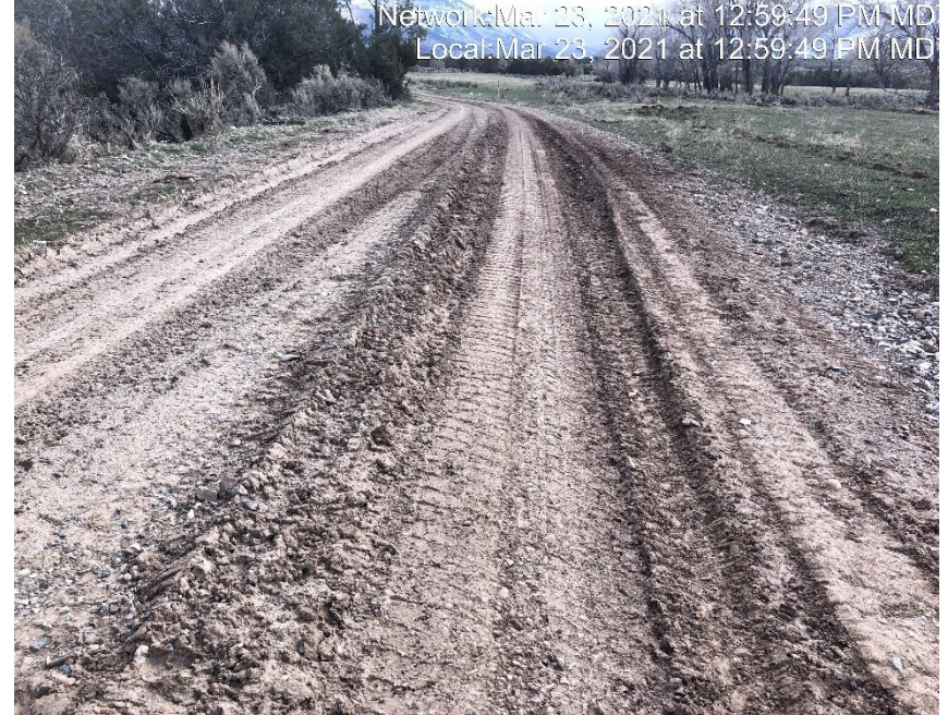
Photo #3250 Access road lacks stabilization
