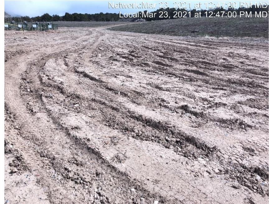
Photo #3244 Location lacks stabilization.
