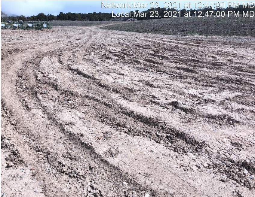
Photo #3243 No form of tracking control
