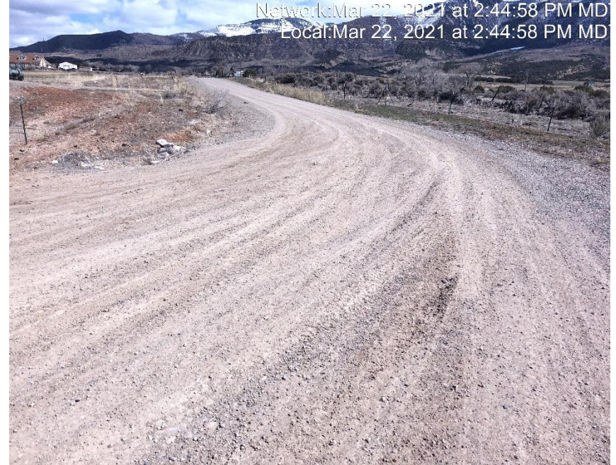
Photo #3236 No form of tracking control at entrance to location
