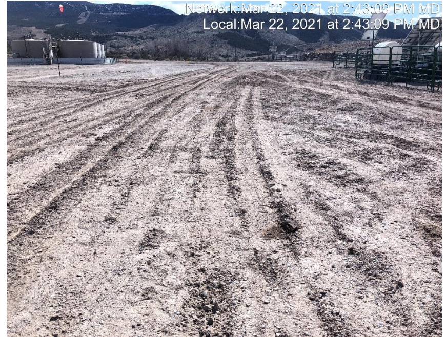
Photo #3234 Location lacks stabilization.
