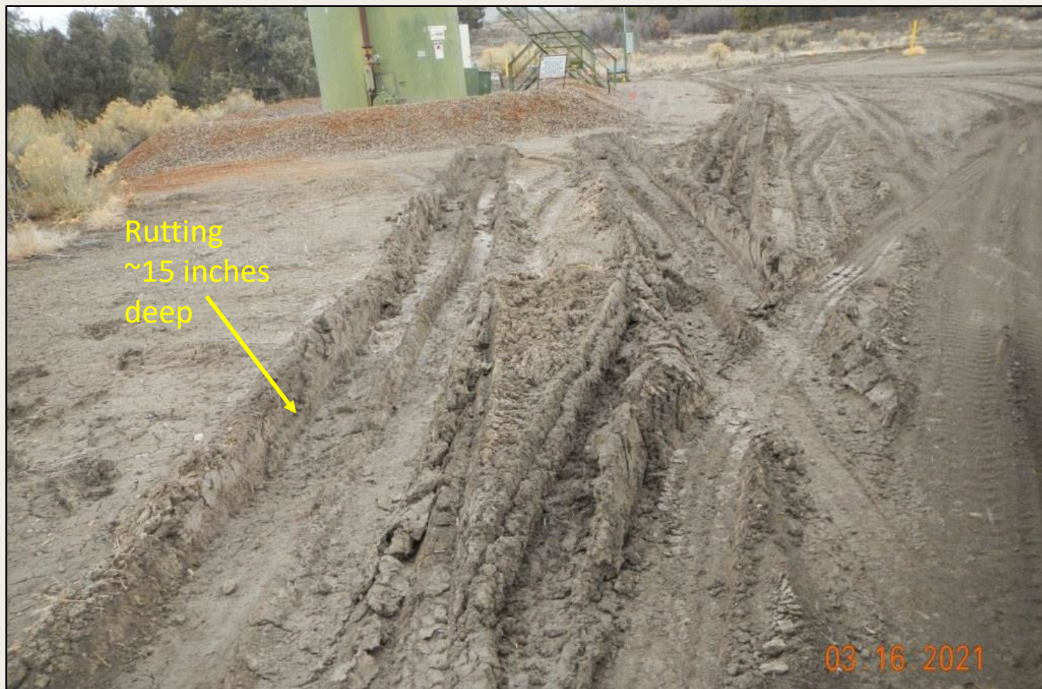
Photo 1. View of deep rutting on the well pad up to approx. 15 inches deep. Stabilization measures need to be installed to prevent site degradation.
