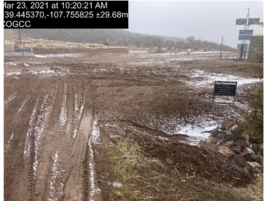
location entrance / Lack of stabilization / compaction
