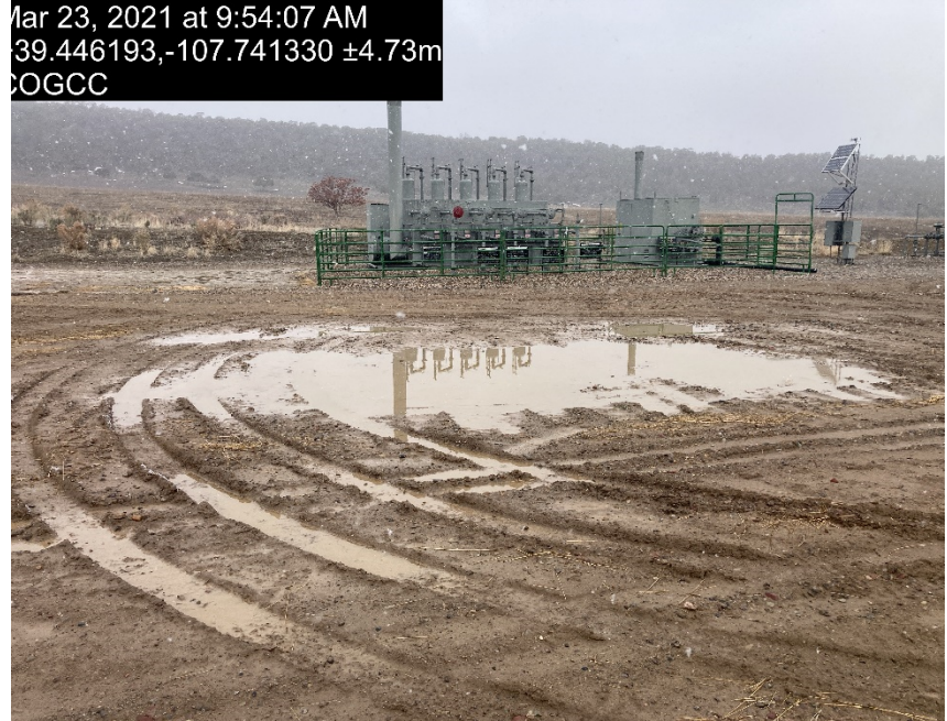
Lack of stabilization / compaction
