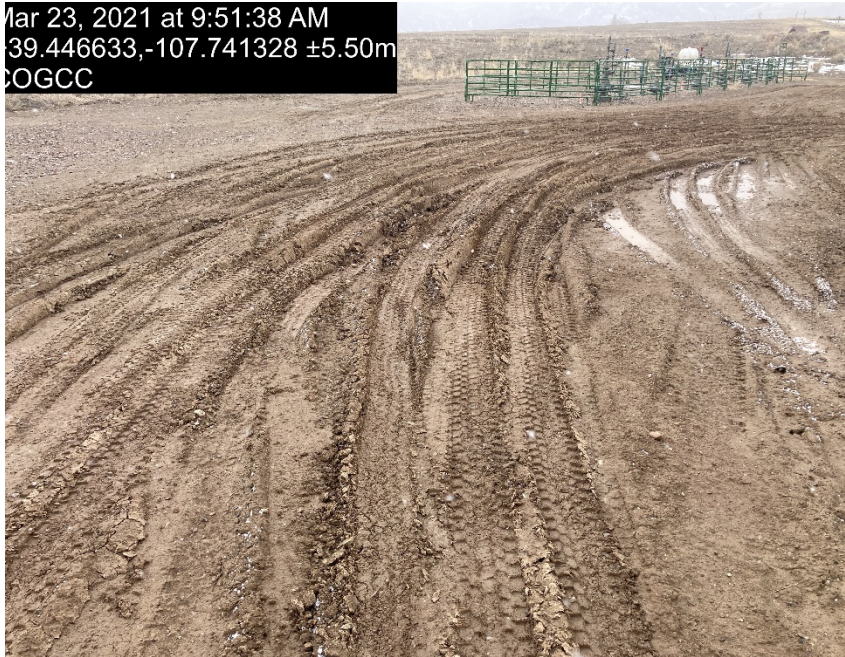
Lack of stabilization / compaction
