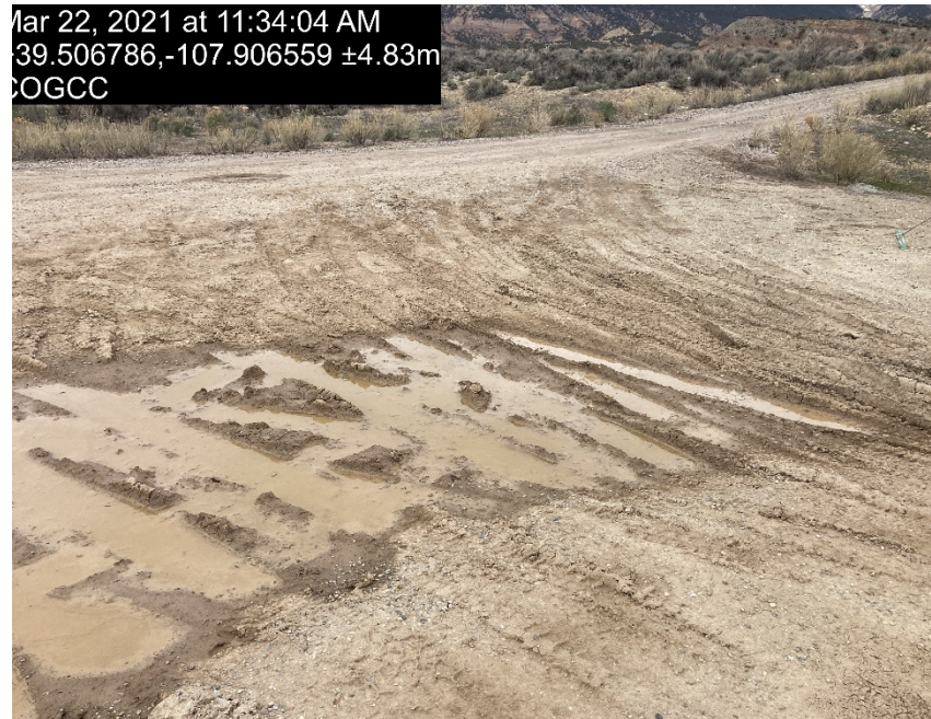
Lack of stabilization/compaction
