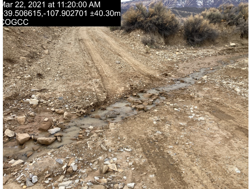
Access road lack of stabilization and drainage crossing
