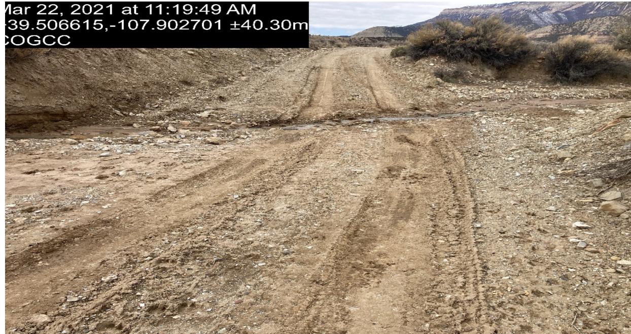
Access road lack of stabilization and drainage crossing
