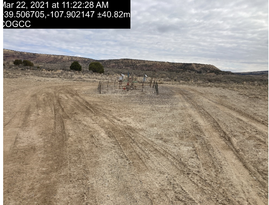
lack of stabilization/compaction on location
