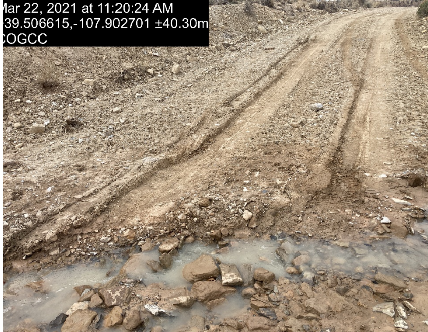
Access road lack of stabilization and drainage crossing
