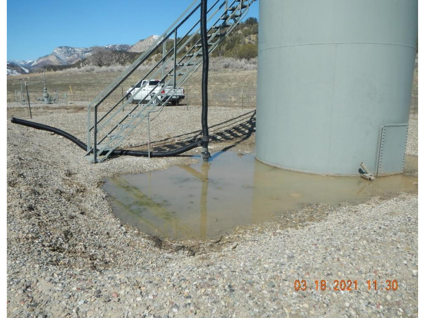
Impoundment of storm water in earthen tank berm.
