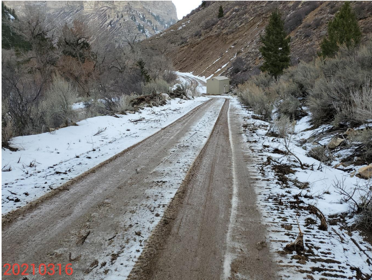
Photo 4: Photo taken from the access road, facing north. Work to reclaim access road pending. Utility pole and shed removed from pad and placed at access road entrance. Equipment requires removal.
