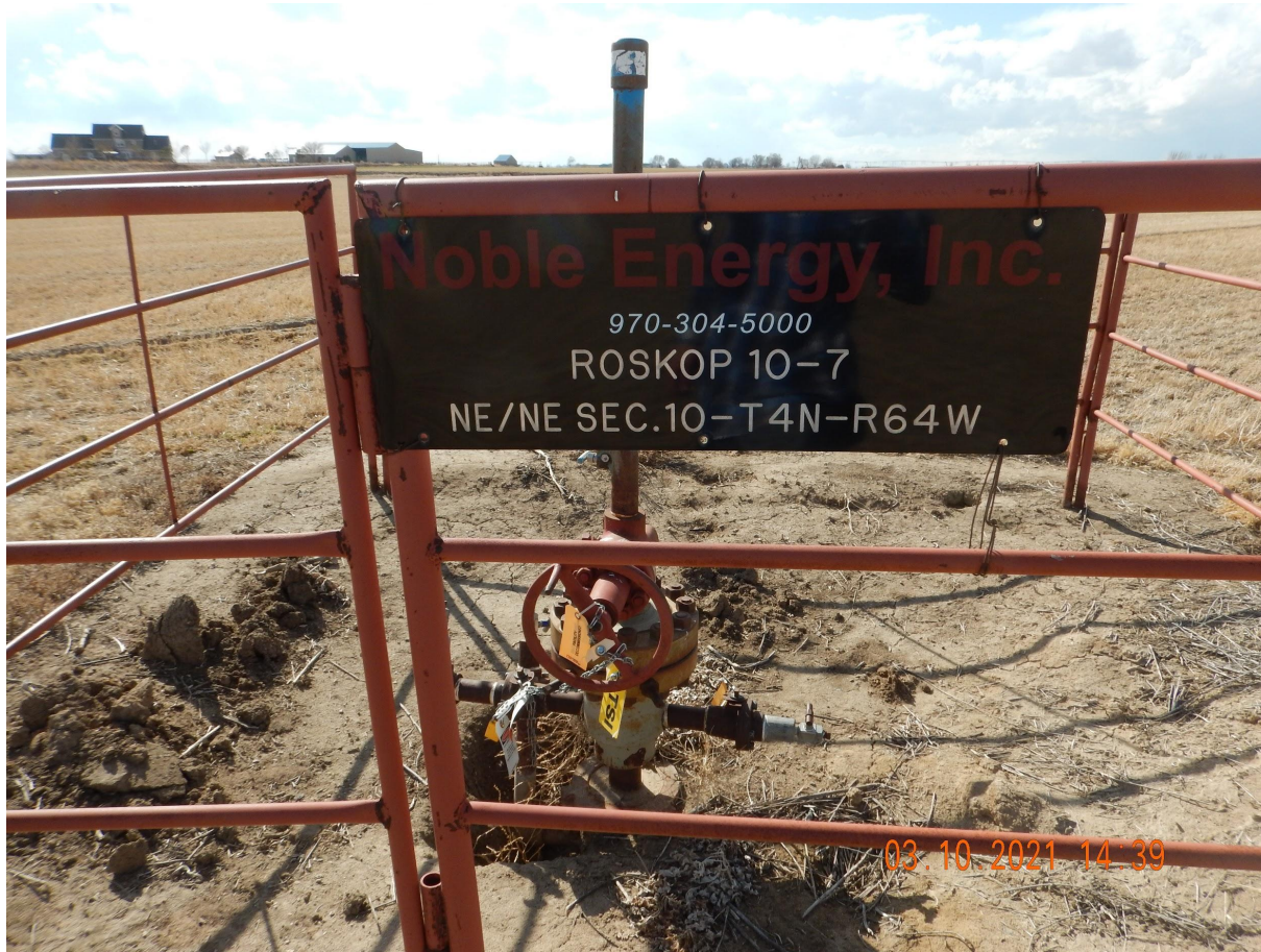
Photo 1. Photo taken from well location. Photo illustrates there are no weed or stormwater issues.
