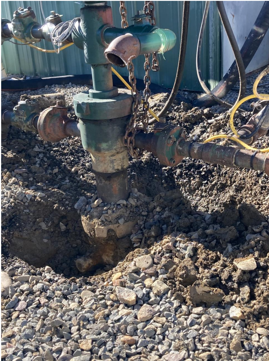
Plumbed bradenhead to surface
