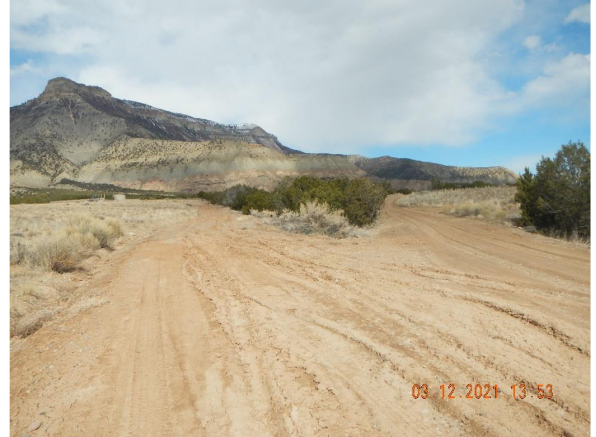
Road lacks stabilization.
