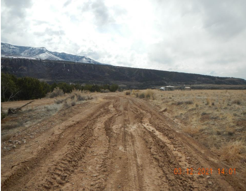
Road lacks stabilization.
