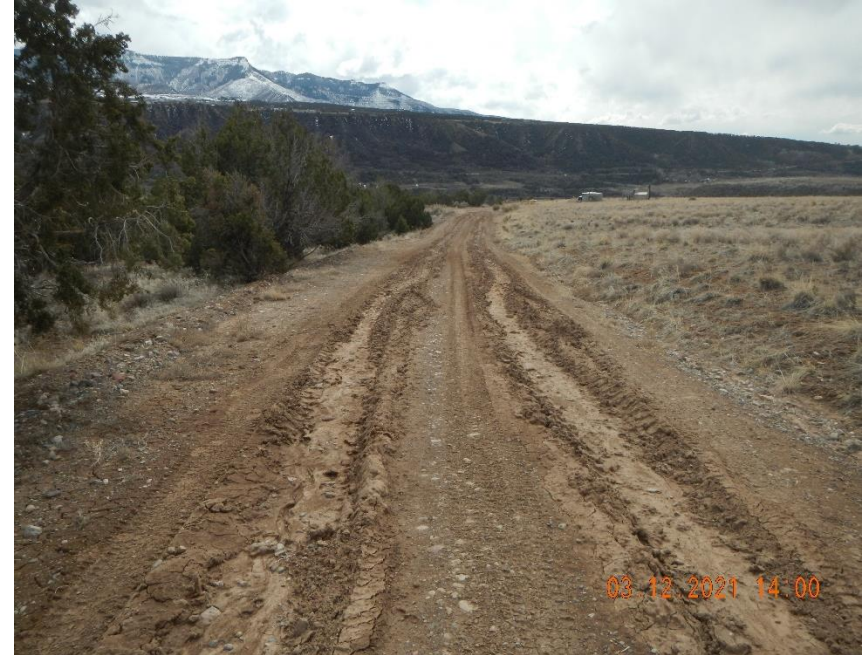
Road lacks stabilization.
