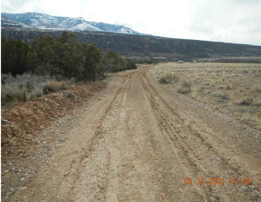
Road lacks stabilization.
