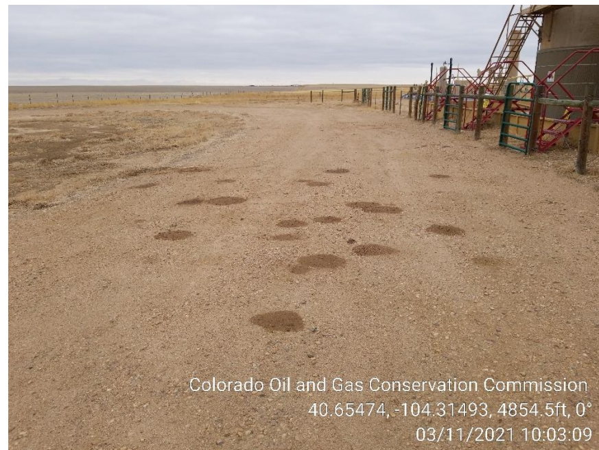
Photo 8 – Stained Soil spots at Tank Battery
