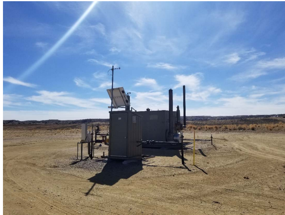
Photo 1. Overview of location taken facing southeast.
