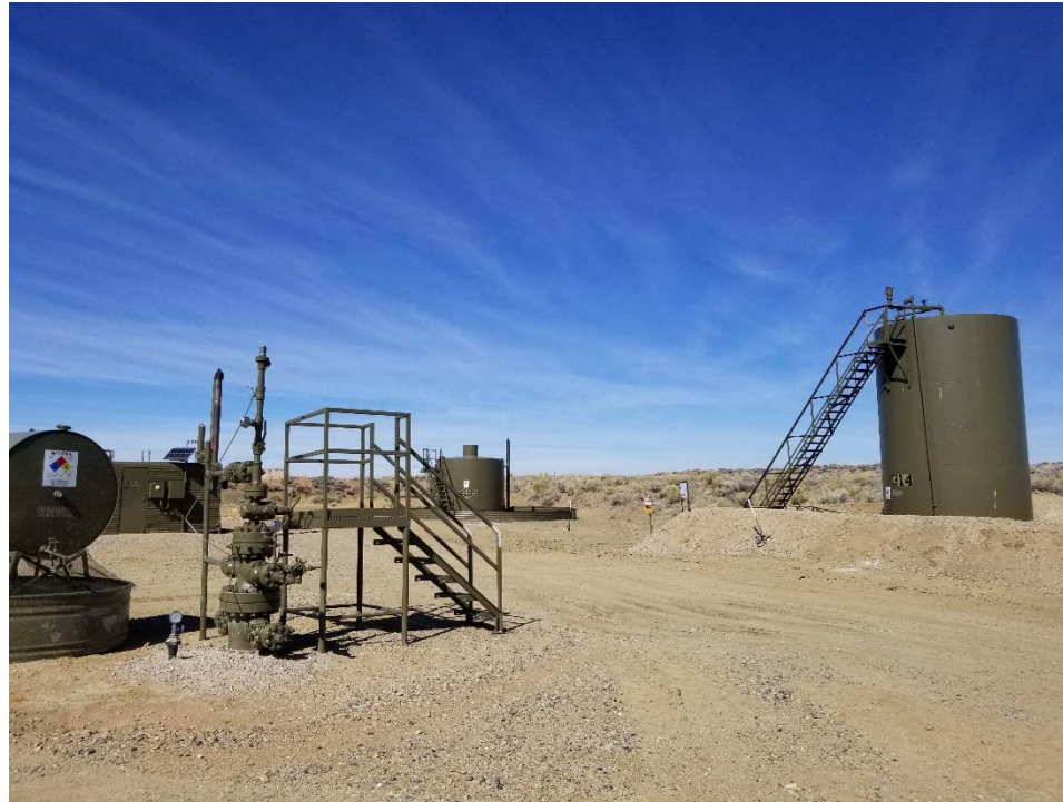
Photo 1. Overview of location taken facing northwest.
