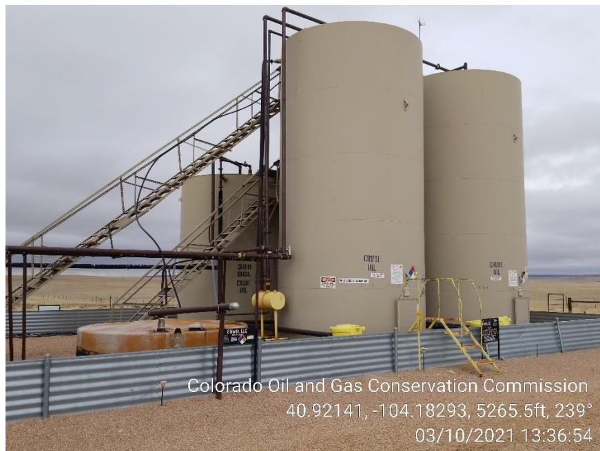
Photo 1 – Tank Battery
