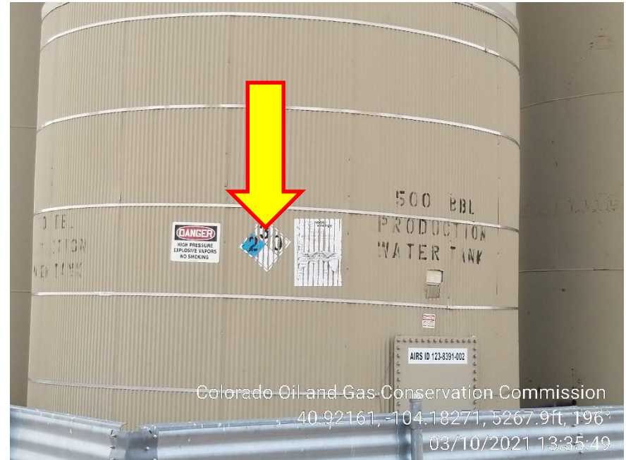
Photo 4 – NFPA Label fading/peeling
