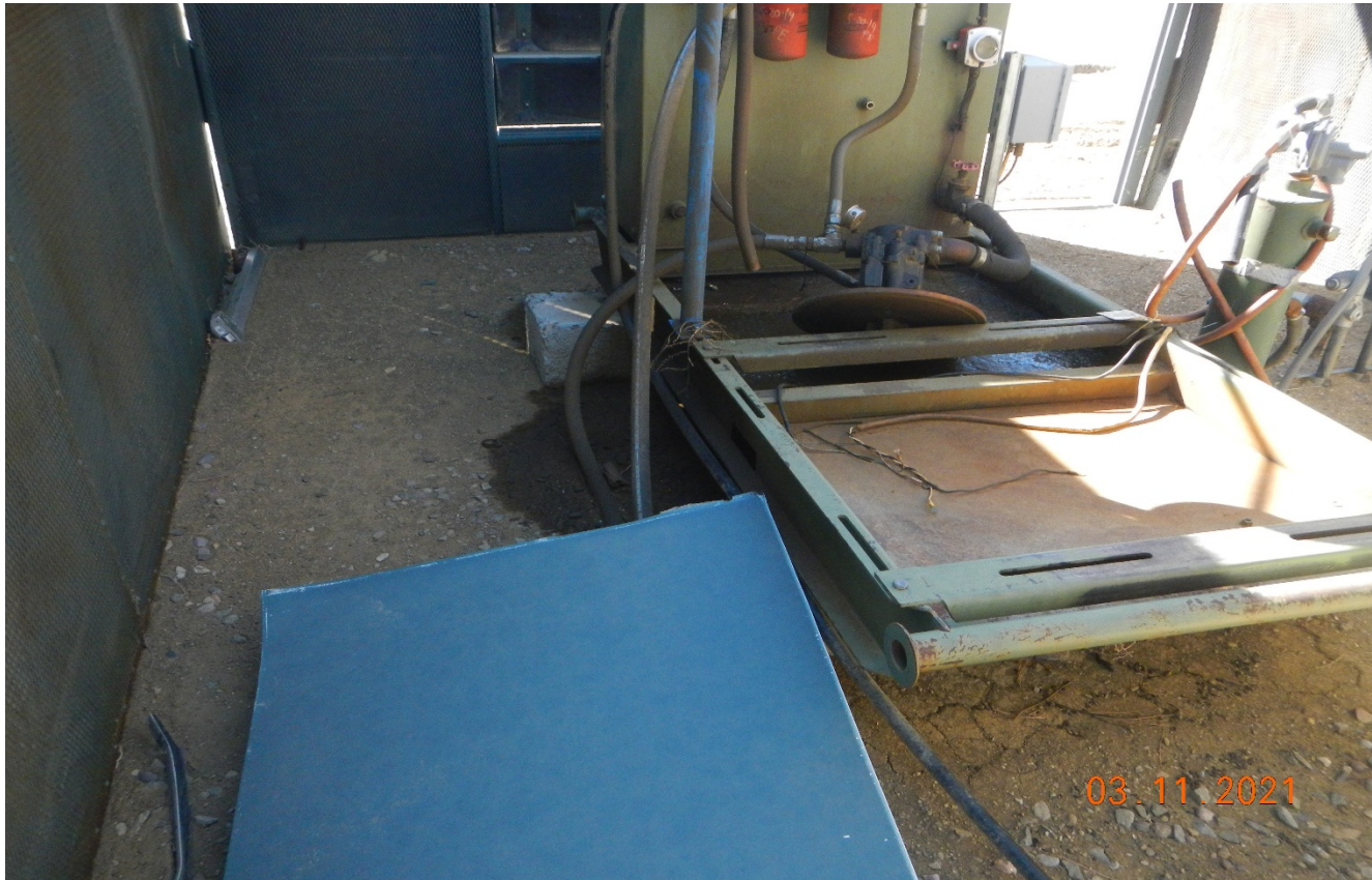
Photo 4. There is oil stained soil under the engine skid.
