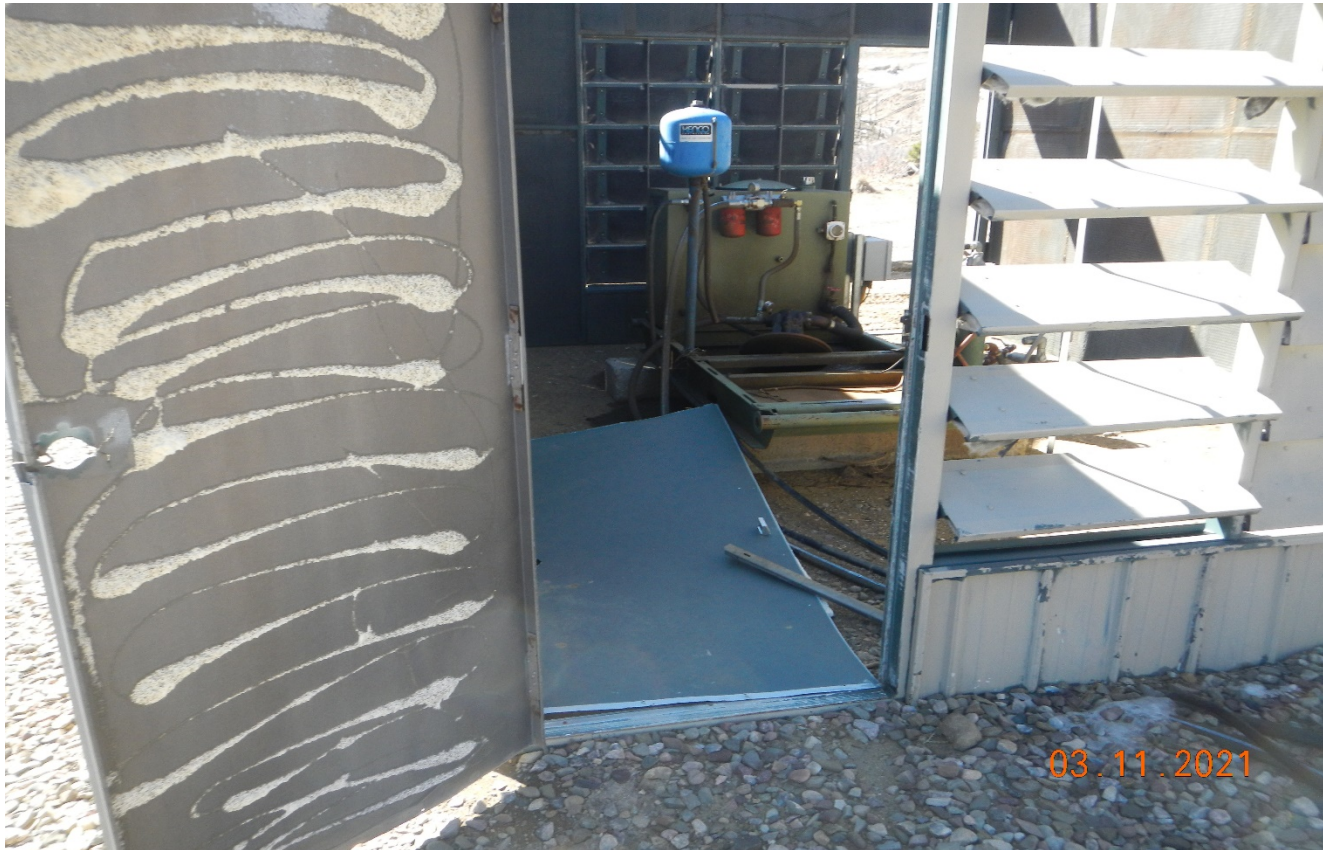
Photo 3. The door on the shed is swinging open. Metal panel laying at entrance way. This need to be repaired or removed.
