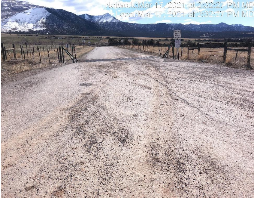
Photo #3180 Sediment has been transported from access road on to county road for approximately 100 yards.
