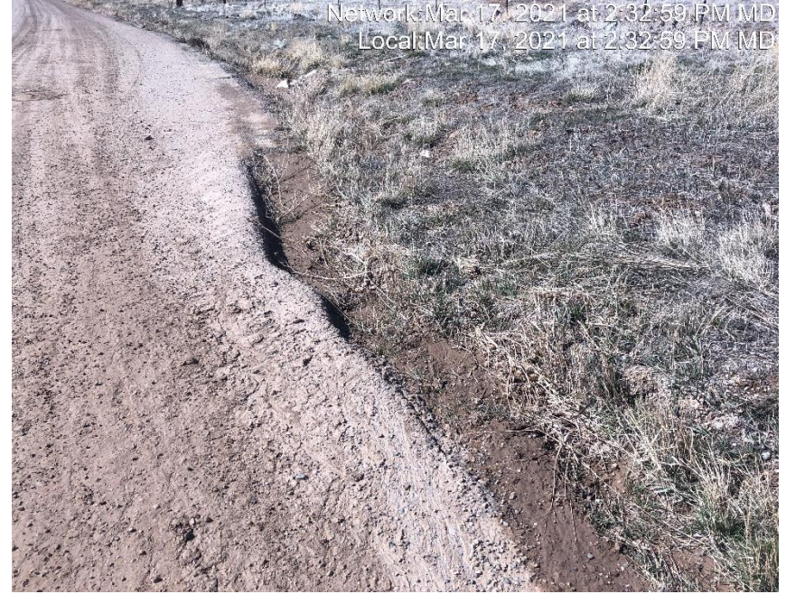
Photo #3181 Sediment from county road has migrated into ditch.
