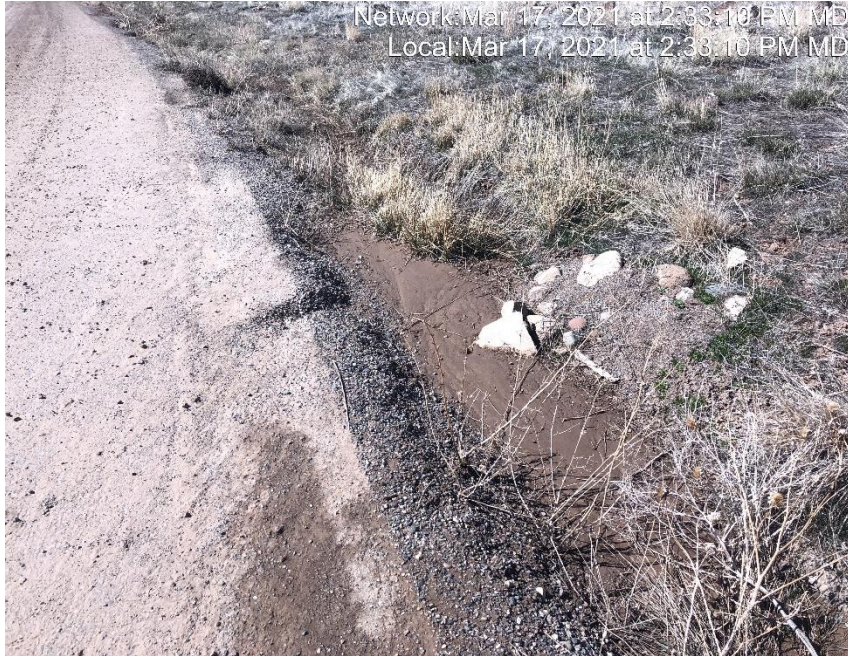
Photo #3182 Sediment from county road has migrated into ditch.
