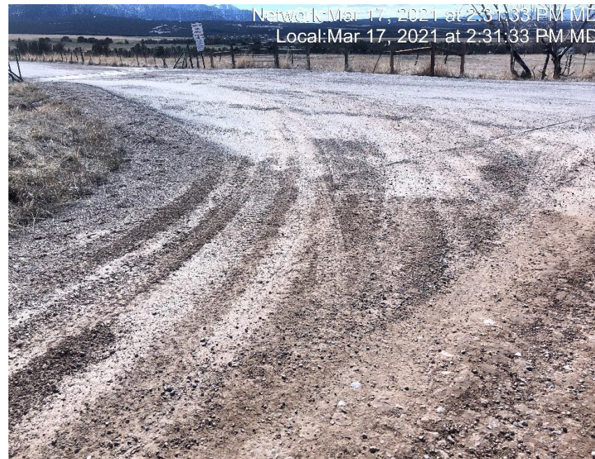
Photo #3177 Tracking occurring from Caerus access road on to county road 306.
