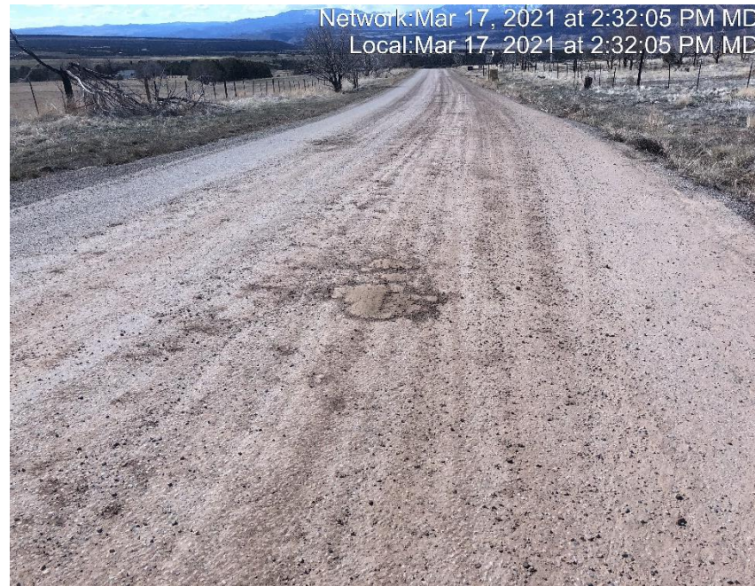
Photo #3179 Sediment has been transported from access road on to county road for approximately 100 yards.
