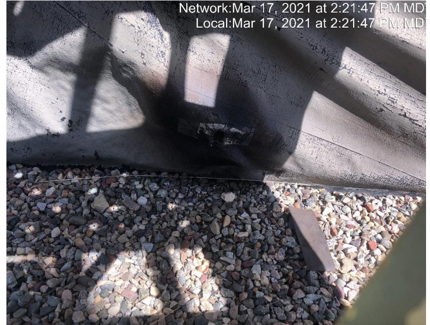
Photo #3173 Multiple holes in tank containment liner.
