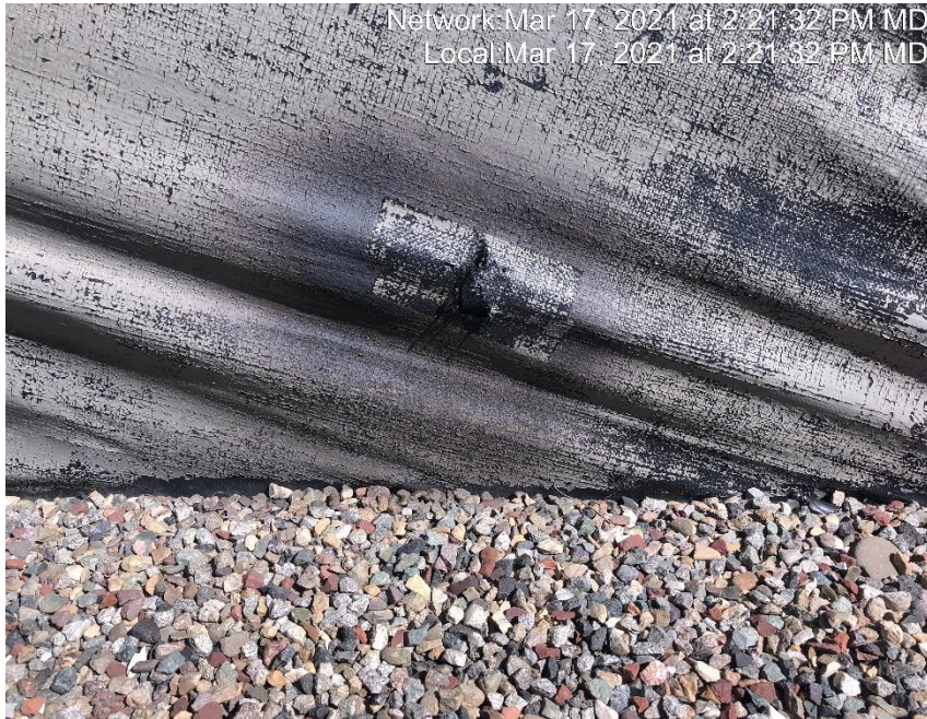
Photo #3172 Multiple holes in tank containment liner.
