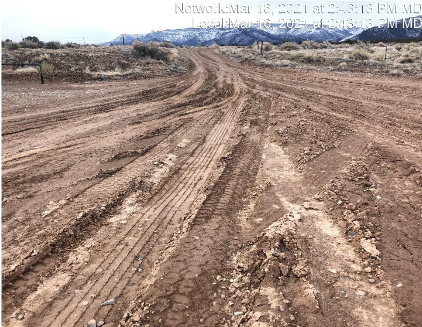
Photo #3166 No form of tracking control at entrance to location.
