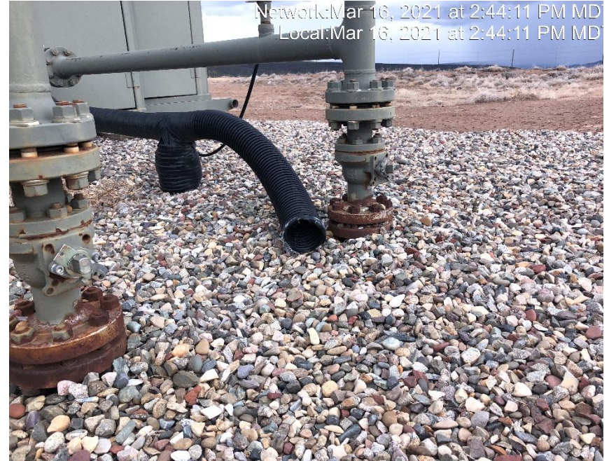
Photo #3167 Flow line heating insulation open ended and not capped.
