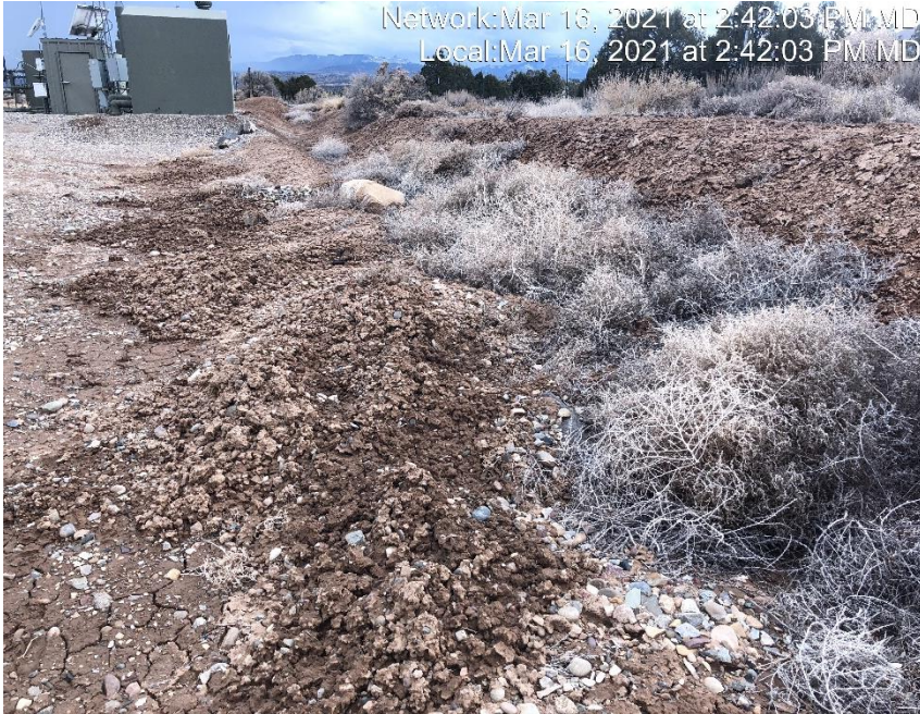
Photo #3164 Sediment appears to have been plowed into ditch
