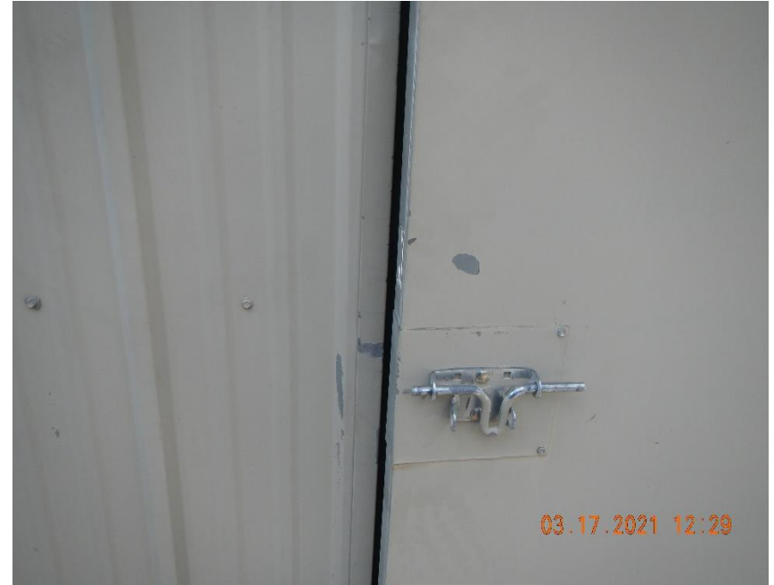
Meter shed door not in working order. No hook for latch.
