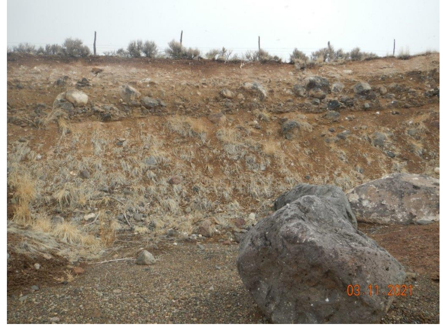
Photo#3: Cut slope at east side of site.
