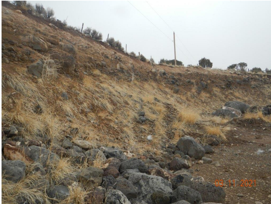
Photo#2: Cut slope at east side of site.
