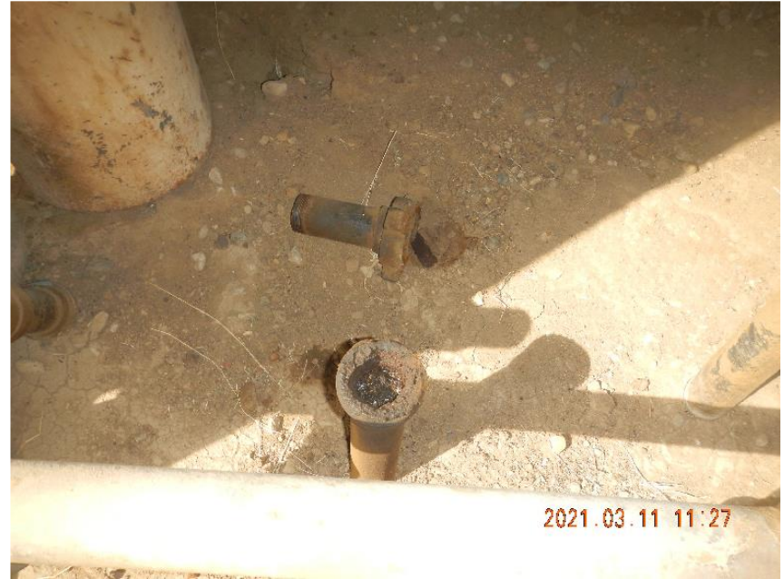
Photo 14: View of open ended riser inside treater shed. Fluid visible inside pipe opening.
