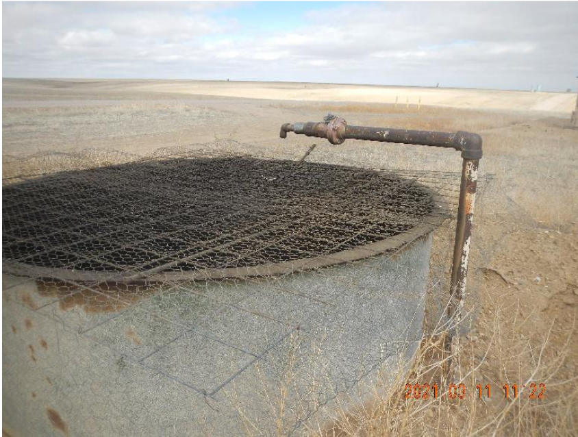
Photo 19: Produced water pit with wildlife screening.
