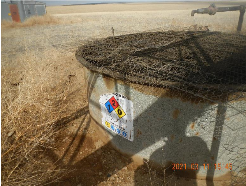
Photo 7: Produced water pit with impacted soil staining around base of pit.
