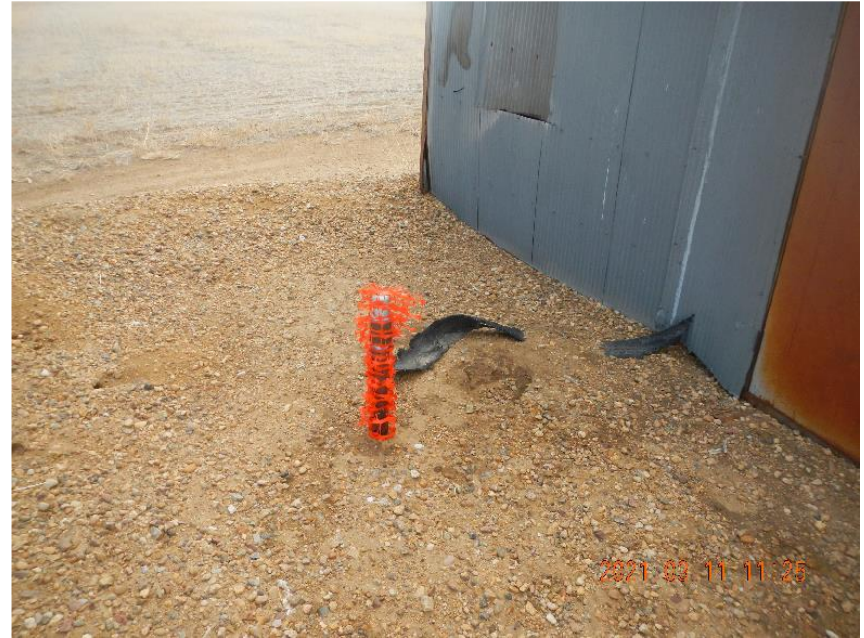
Photo 10: View of plugged riser outside treater shed.
