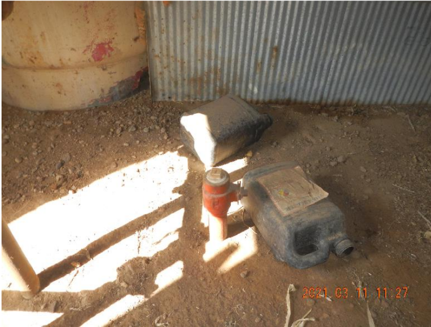
Photo 13: Plugged riser inside treater shed.
