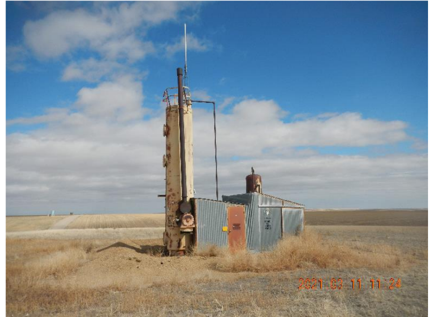
Photo 8: View of vertical heater treater, treater shed, and vertical separator.
