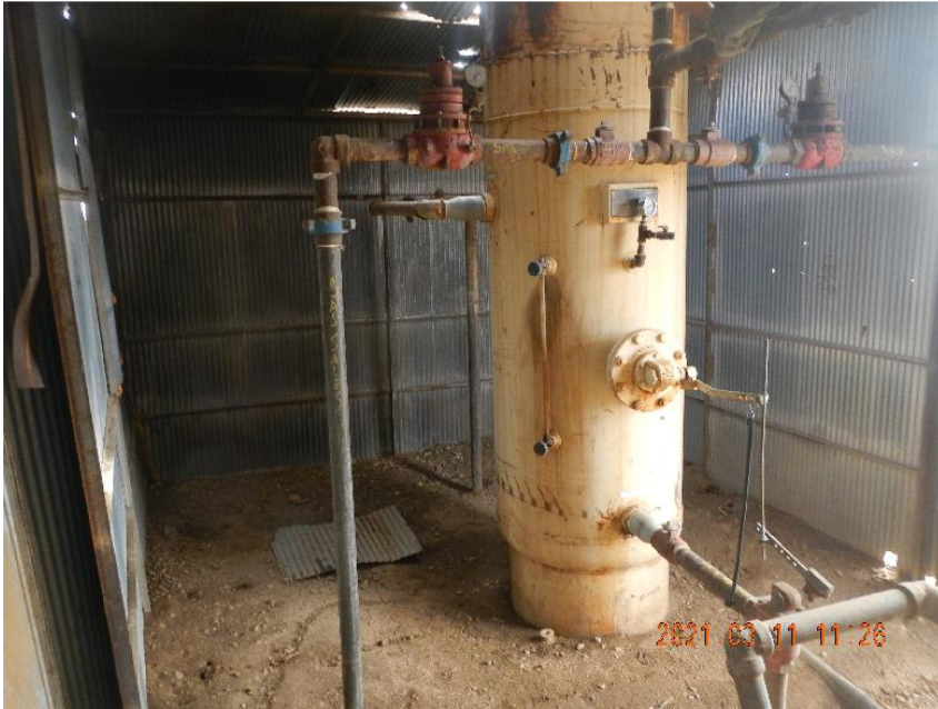
Photo 11: Vertical separator inside treater shed.
