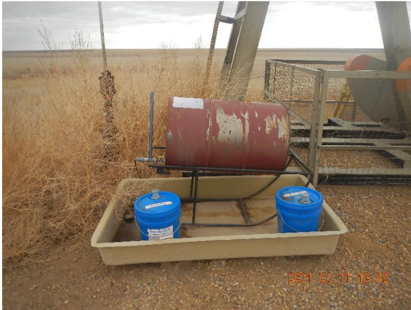
Photo 7: Chemical tank and containment at well site. Two of four 5 gallon buckets.
