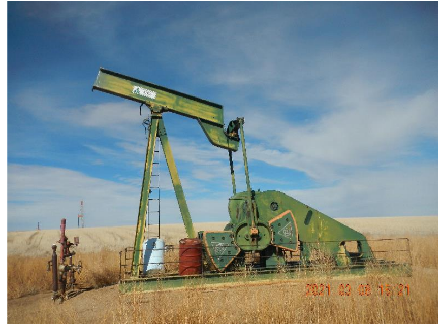
Photo 10: View of unused pumping unit with horsehead removed.
