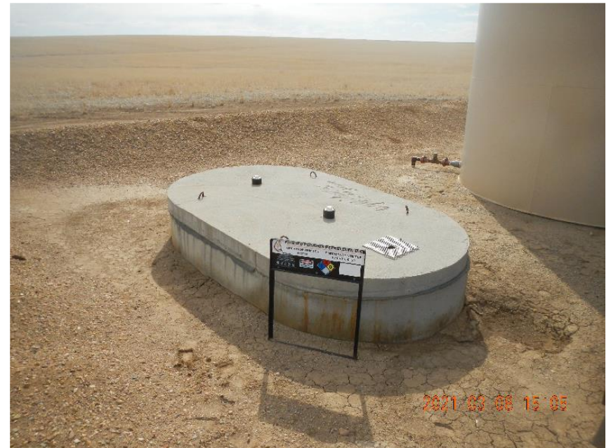
Photo 4: 48 BBL concrete pit.
