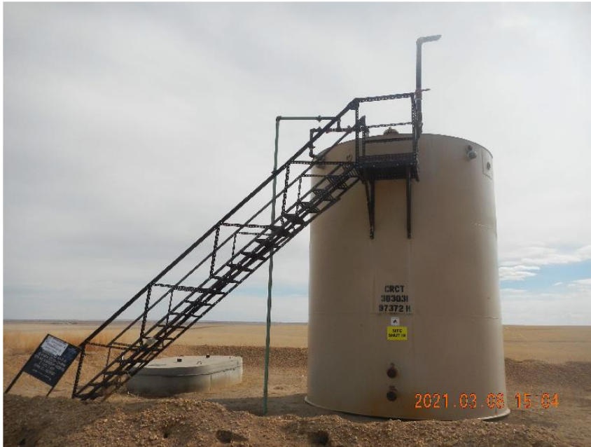
Photo 3: 300 BBL steel tank.
