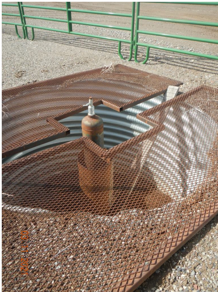
Photo#4: Escape Boards in cellars not adjusted properly.
