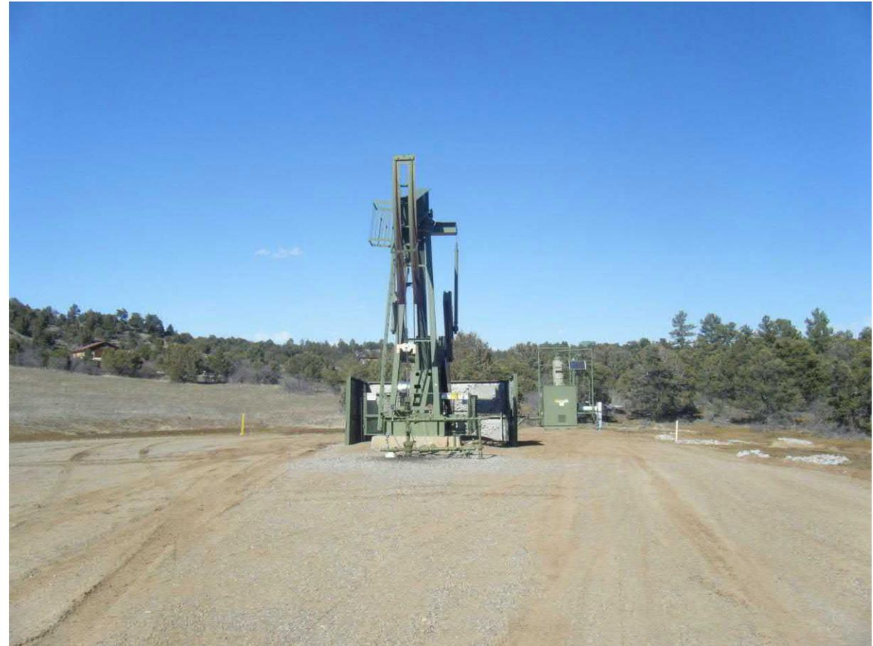
Storm Water management controls have been installed and re-established to stabilize erosion. Re-established drainage diversion on the east side of pad. Re-contoured drainage, repaired erosion cuts, installed silt traps, and rock rundowns to de-energize storm water run off. Spot seeded disturbed and barked areas on southeastern fill slope.
