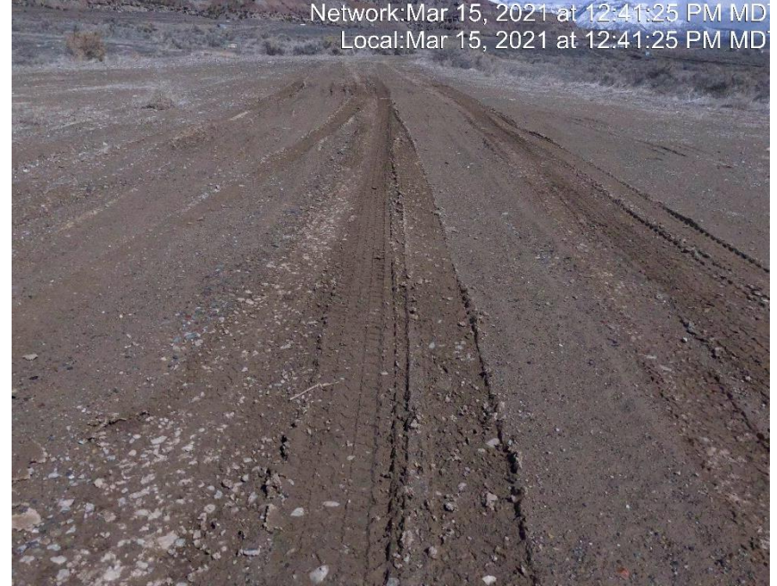
Photo #3142 No form of tracking control at entrance to location.
