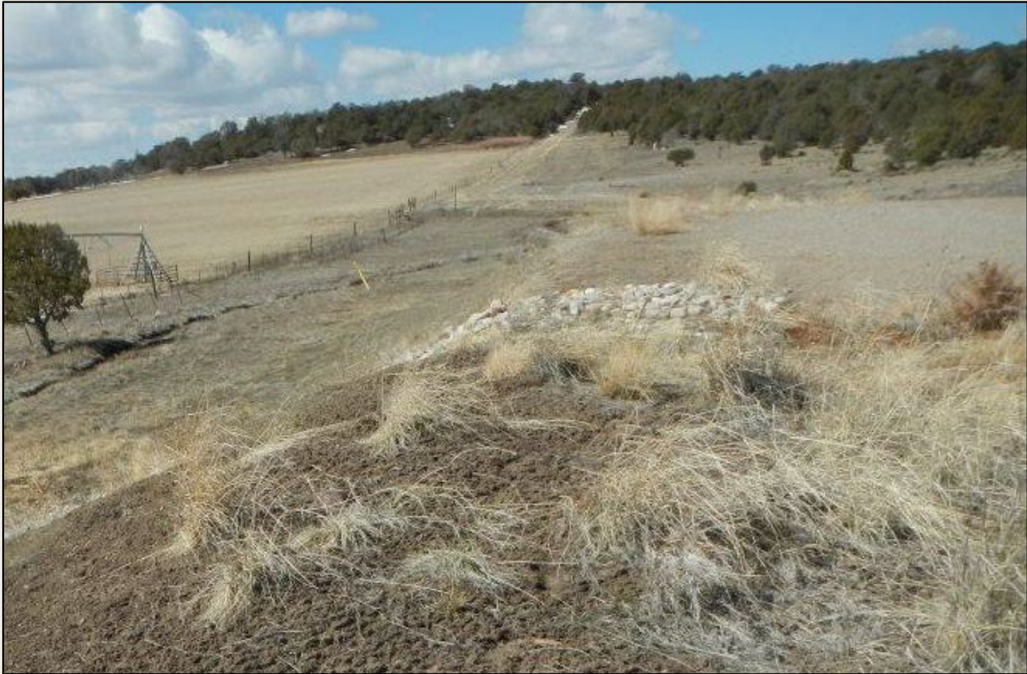
Photo 2. View of the southern project area from the southeastern corner facing westward. Sparse revegetation observed in portions of the fill slope where spot seeding may be needed.
